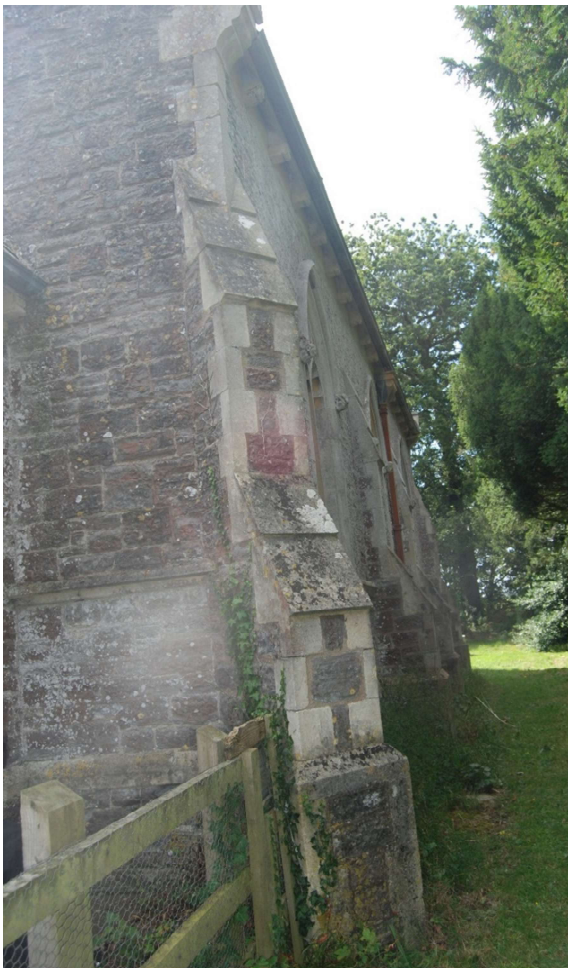
Figure 66 South aisle looking west
