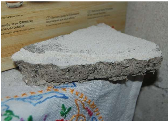
Figure 10 Fragment of mortar from the internal vestry wall.
