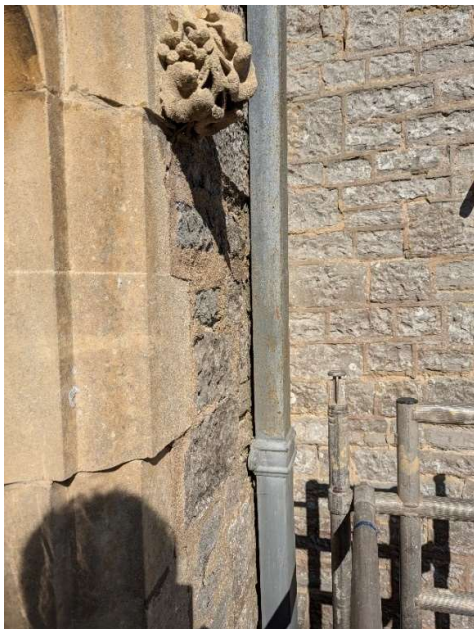
Figure 49 Displacement of east jamb at mid height
