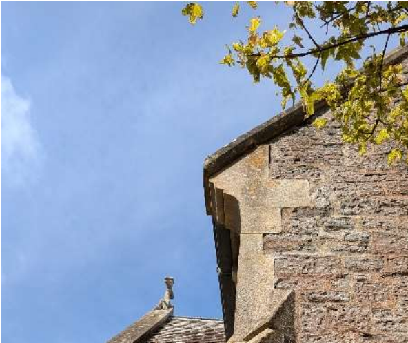
Figure 58 Opening of upper south corner of the chancel east gable
