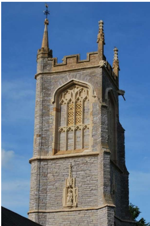
Figure 79 Example of lias consolidation and repair to St Michael's Church, Othery.
