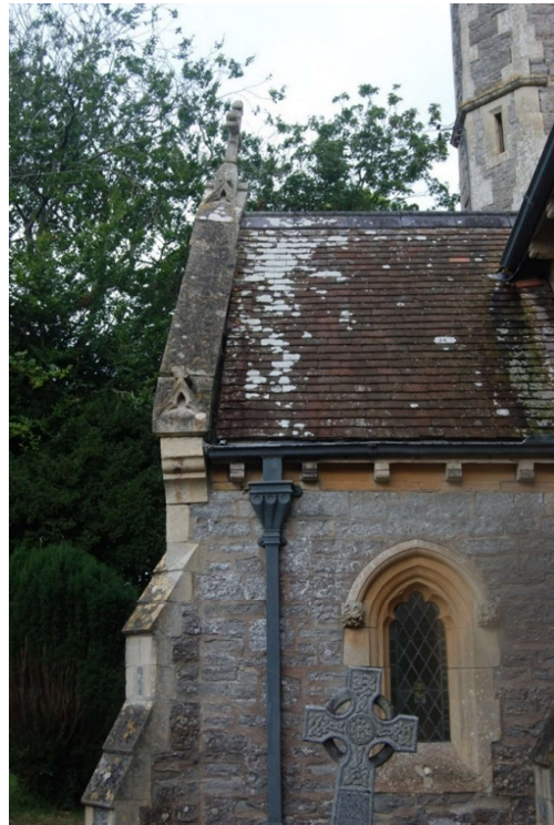
Figure 33 South porch gable from the east
