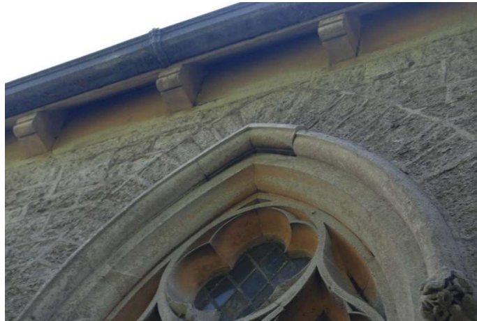
Figure 71 Displacement of the key stone
