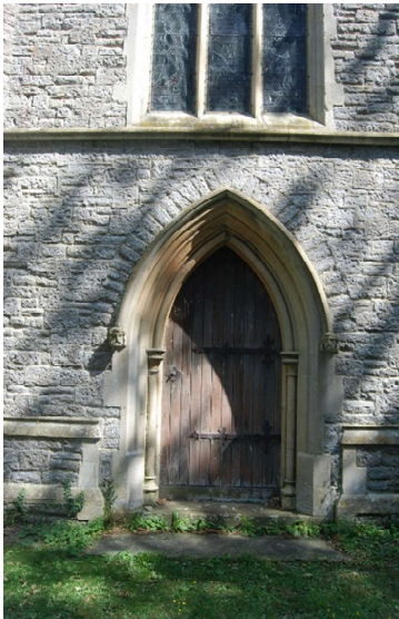
Figure 76 Tower west door
