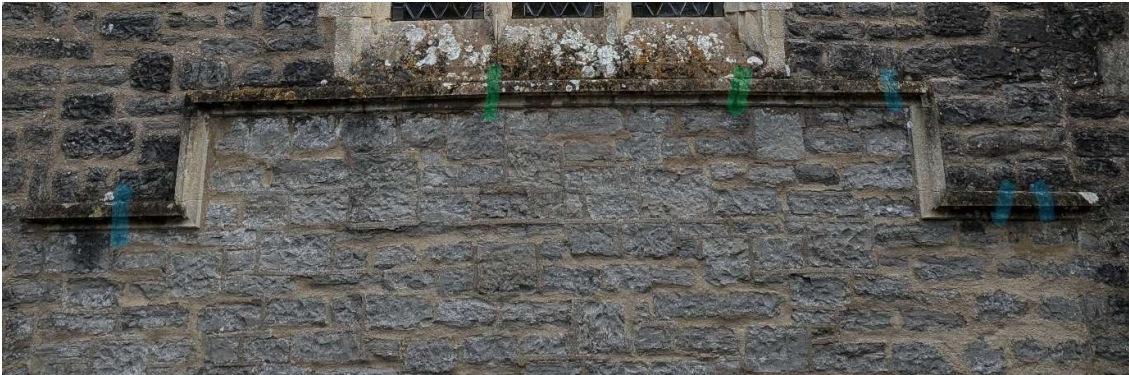
Figure 53 Rising and falling of the string course beneath the window
