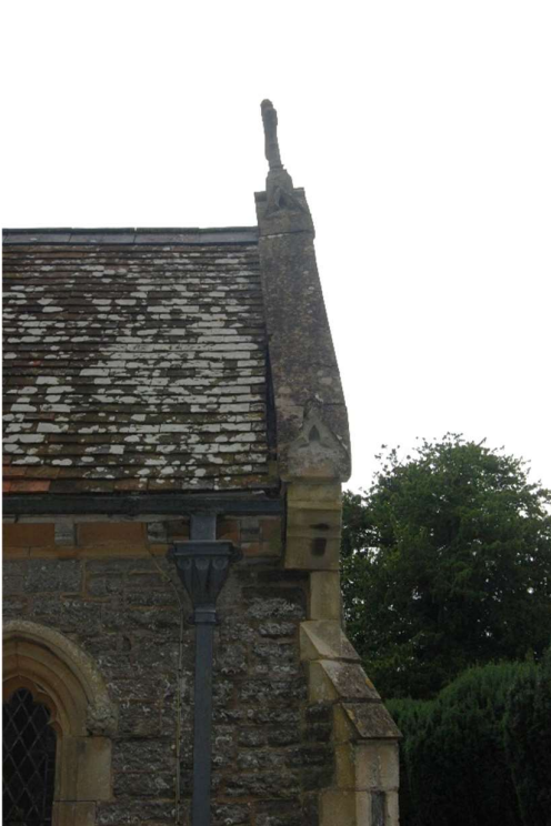
Figure 32 South porch gable from the west
