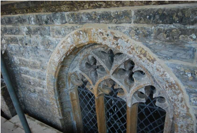
Figure 78 Example of Blue Lias and Ham stone repair and repointing at Low Ham Church
