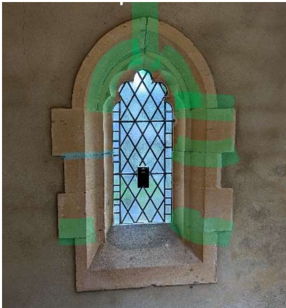
Figure 34 South porch east window internal face
