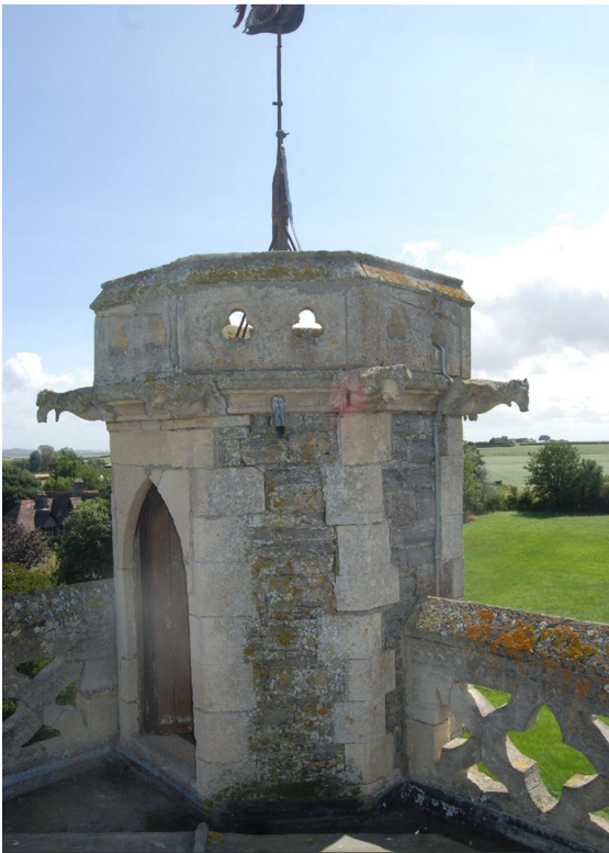
Figure 22 The vice turret viewed from the north west.
