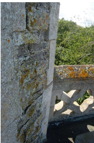
Figure 24 Weathered blue lias surface to the vice turret on the north west side.
