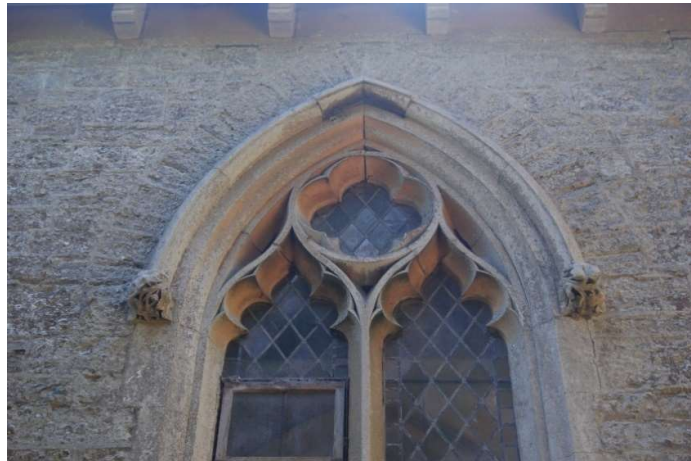
Figure 74 Displaced keystone
