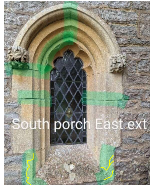
Figure 35 South porch east window external face
