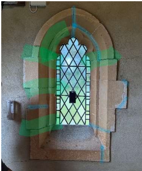
Figure 38 South porch west window internal face
