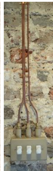
Legacy gas lamps and pipework on piers at St. Mary Magdalene; Examples of Mineral Insulated Copper Cable (MICC) specified by MF in heritage buildings: (St. Mary Magdalene church, Paddington), (Wiltons Music Hall)
