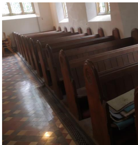
Apply Insulation to floors
