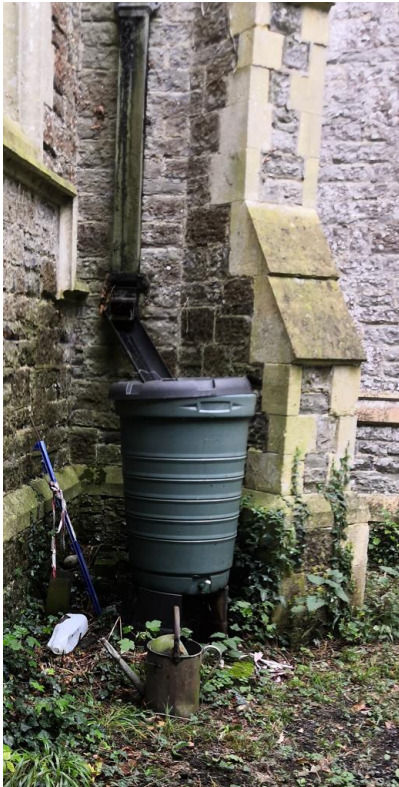
Existing water butt at the back of the Church
