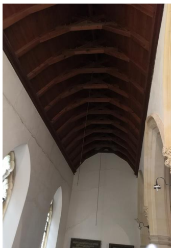
Apply insulation to roof
