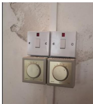
Existing 180W under-pew direct electric heaters with dual zone wall control
