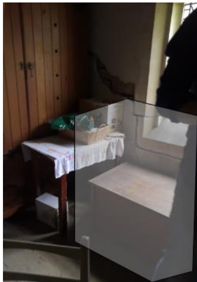
Area of the Vestry where new Accessible WC is to be introduced
