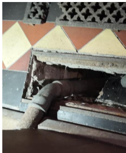
Old cast-iron radiators and pipework running in trenches
