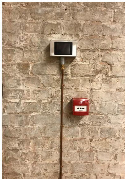
Legacy gas lamps and pipework on piers at St. Mary Magdalene; Examples of Mineral Insulated Copper Cable (MICC) specified by MF in heritage buildings: (St. Mary Magdalene church, Paddington), (Wiltons Music Hall)
