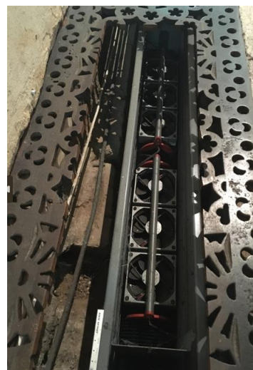
Fan-Assisted Trench Heaters
