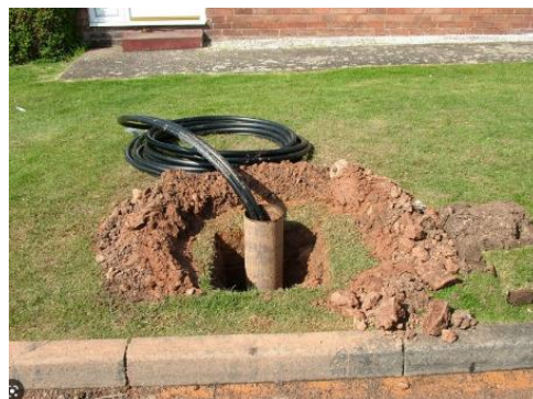
Ground Source Heat Pump (Vertical)
