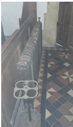
Old cast-iron radiators and pipework running in trenches
