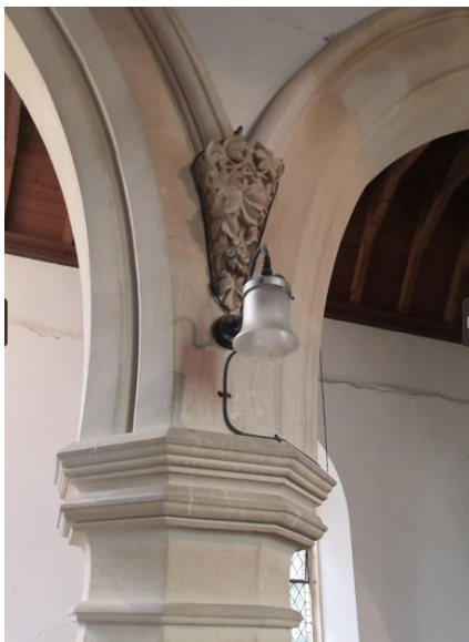
Legacy gas lamps and pipework on piers at St. Mary Magdalene; Examples of Mineral Insulated Copper Cable (MICC) specified by MF in heritage buildings: (St. Mary Magdalene church, Paddington), (Wiltons Music Hall)
