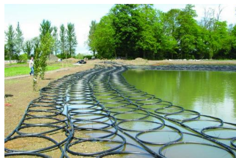
Water Source Heat Pump
