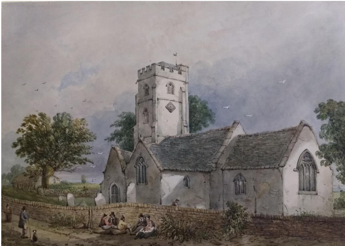
Original St Mary Magdalene before demolition as per print in vestry.
