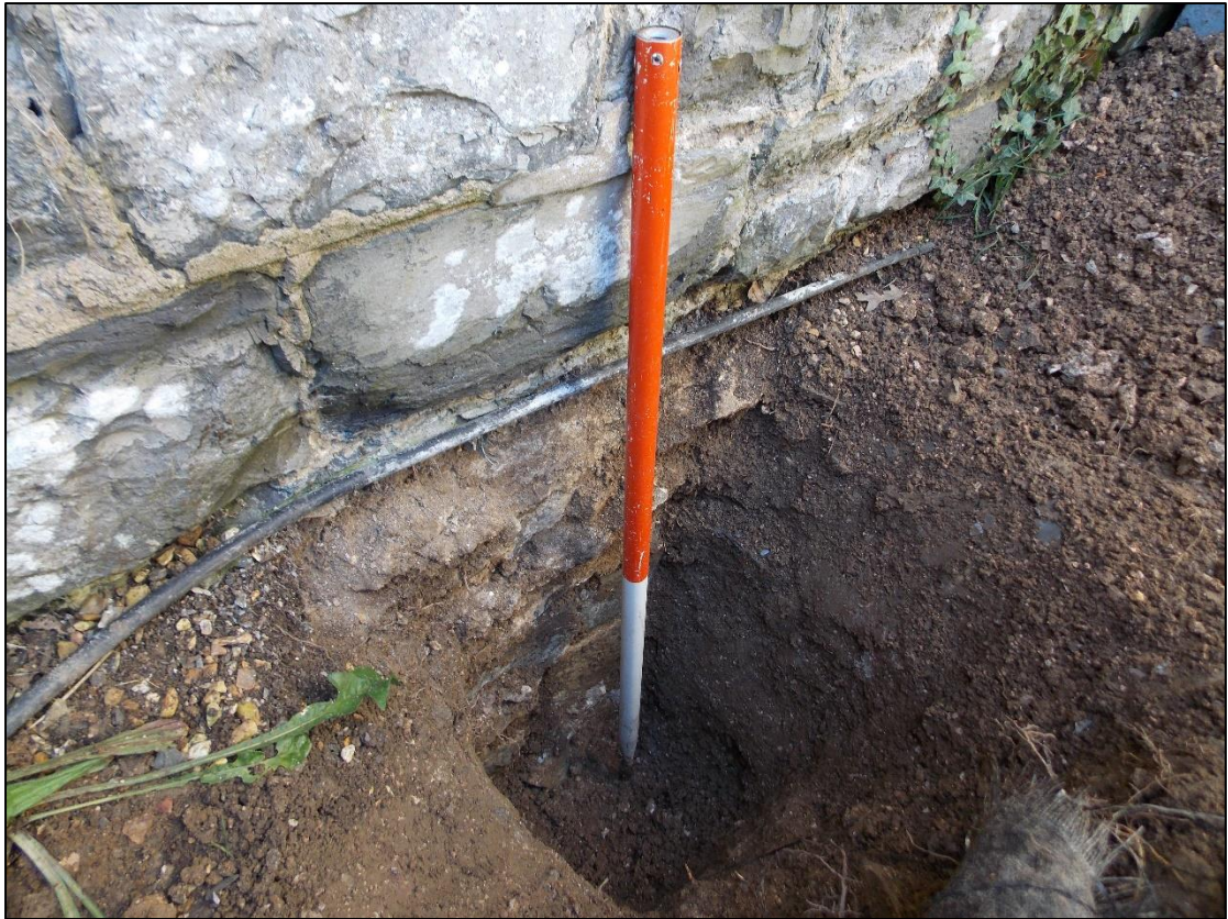
Figure 5. TH2: facing NW, 1m scale.
