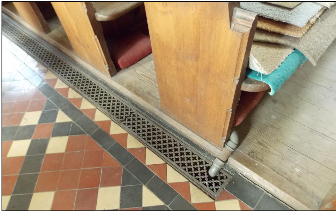
Figure 12. Service duct at east end of pews: facing NW
