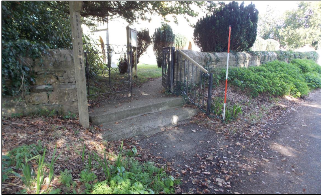
Figure 8. Stepped gateway entrance: facing NE, 2m scale
