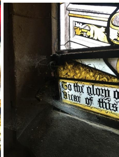
Bowing of lead work caused by movement of jamb stones- detail of seized sill casement
