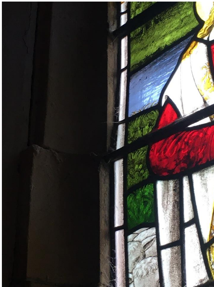
Bowing of lead work caused by movement of jamb stones- detail of seized sill casement
