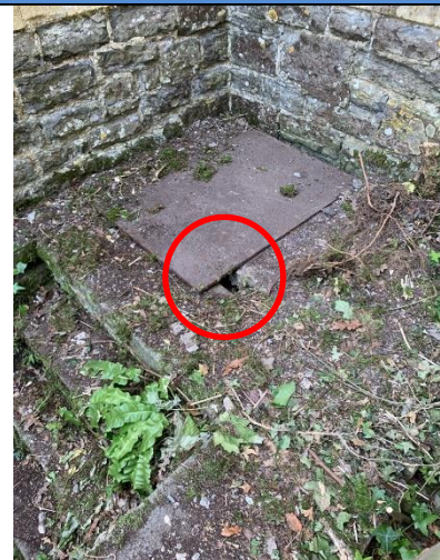
4.24 Disused coal chute into the boiler room. Red circle indicates potential bat access point.
