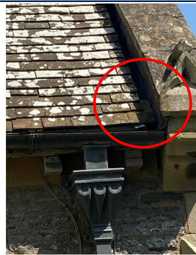
4.28 Lifting leadwork around edge of tiles. Red circle indicates potential bat access point.
