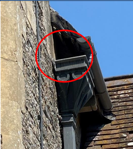
4.27 Rotten soffit board above drain. Red circle indicates likely bat access point.
