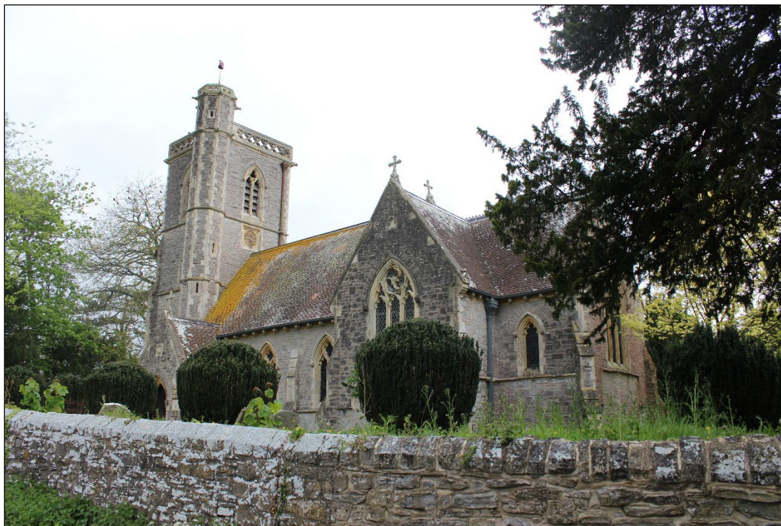
Above: The church viewed from the road.
