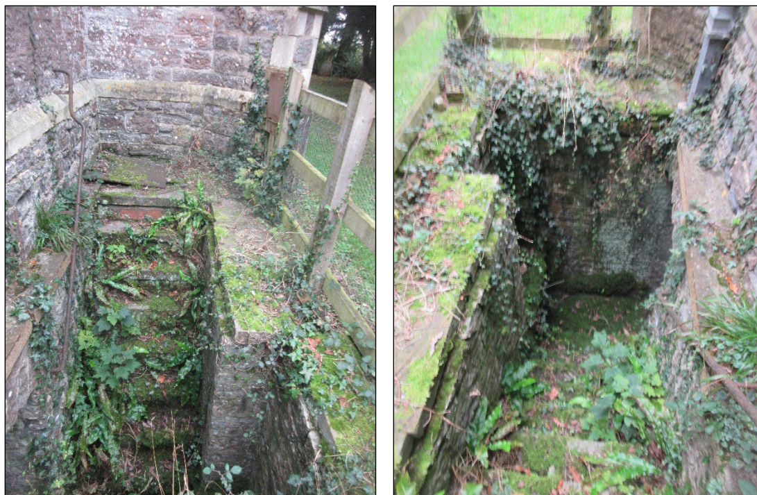
Above: Photos of the existing boiler room stair and fencing.
