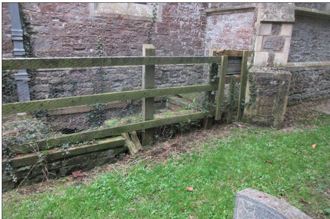
Above: The existing post and rail fencing with chicken wire.
