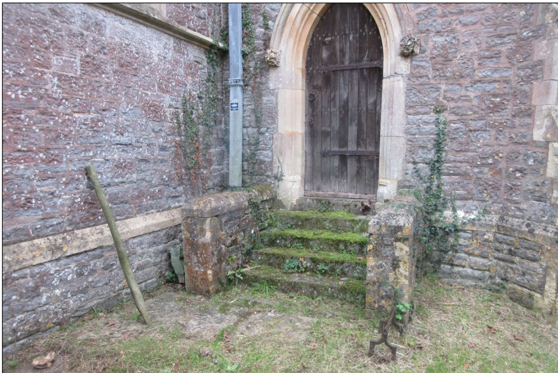
Above: The existing steps up to the vestry.
