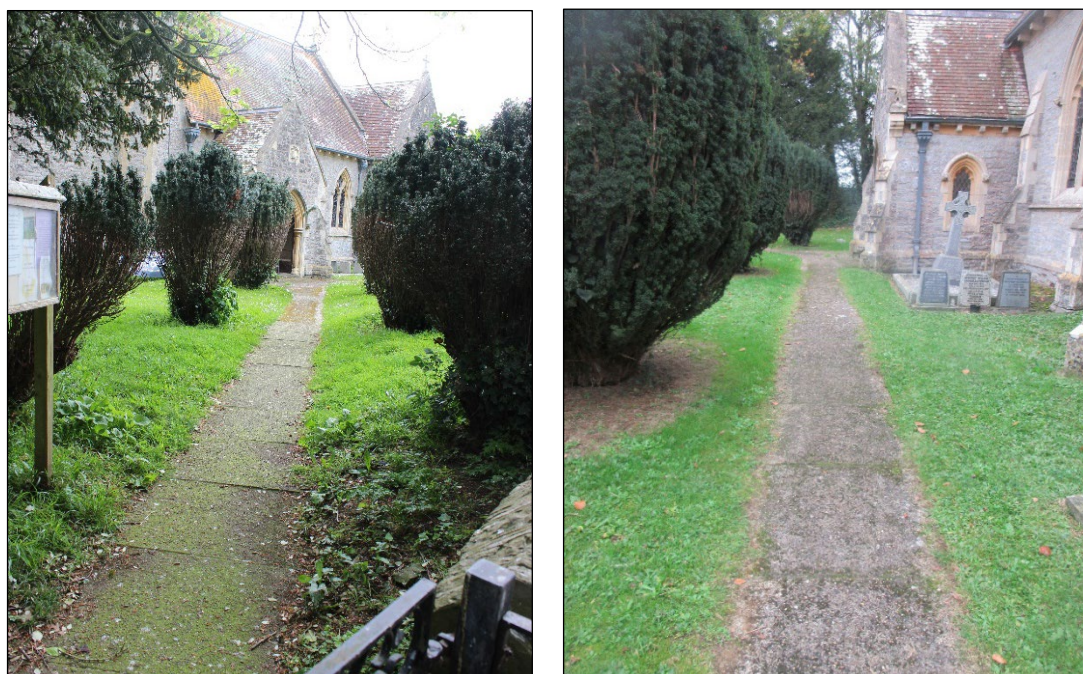
Above: The existing concrete paths is laid with slabs which will be lifted and relaid.
