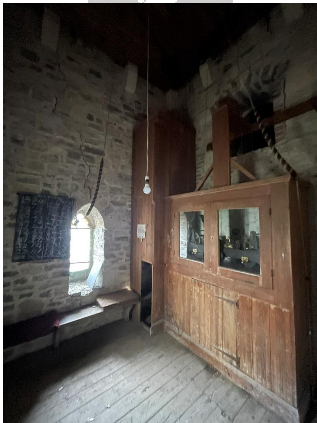
The first-floor ringing chamber showing the clock case and weight chute.
