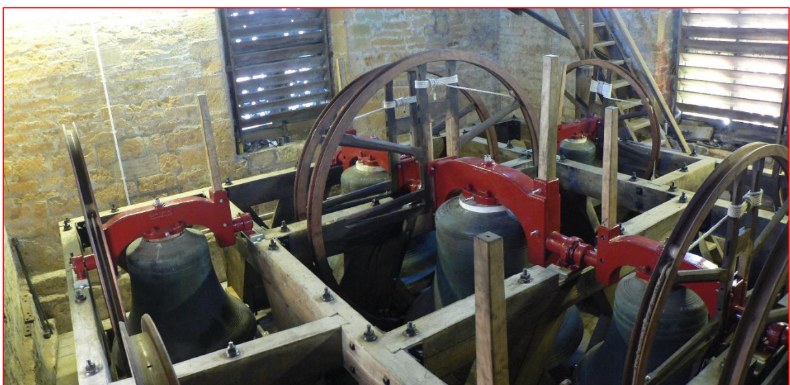
Photo: Milborne Port bells rehung with all new fittings in their existing bellframe
