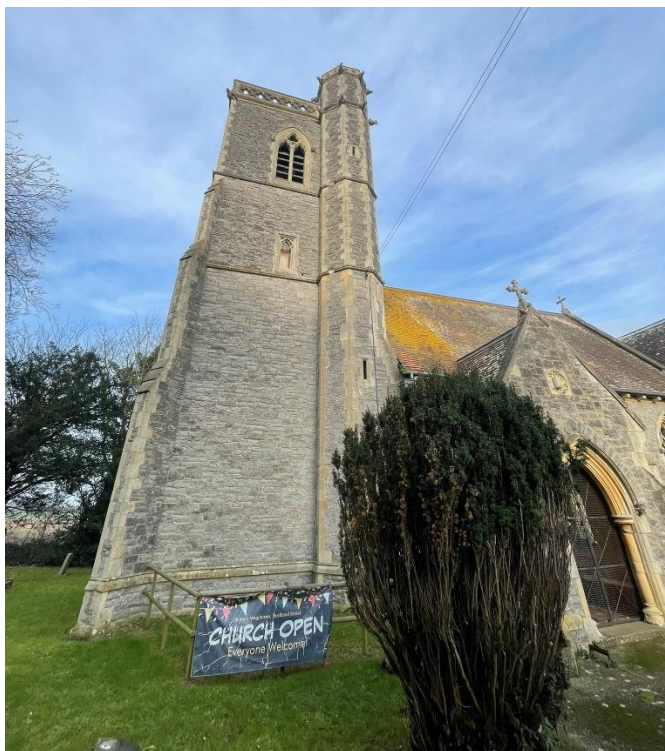
The tower from the south.
