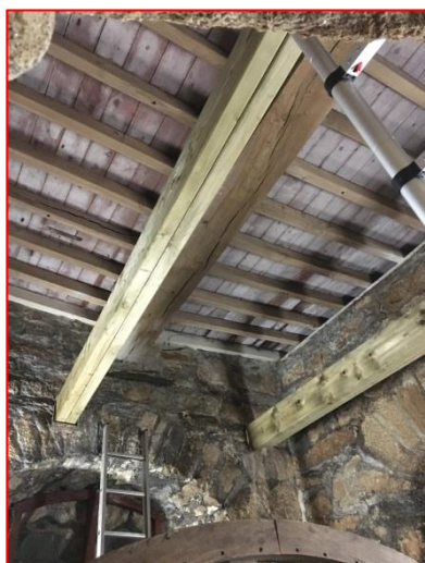
Photo: Typical arrangement of temporary lifting beams (where there are no fixed roof beams in position to lift from).
