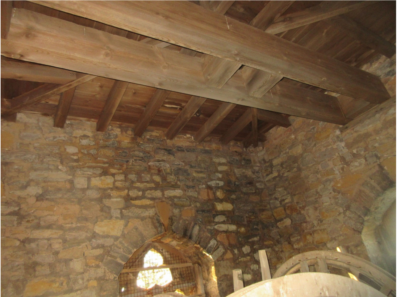
Above: The Bell Chamber ceiling.
