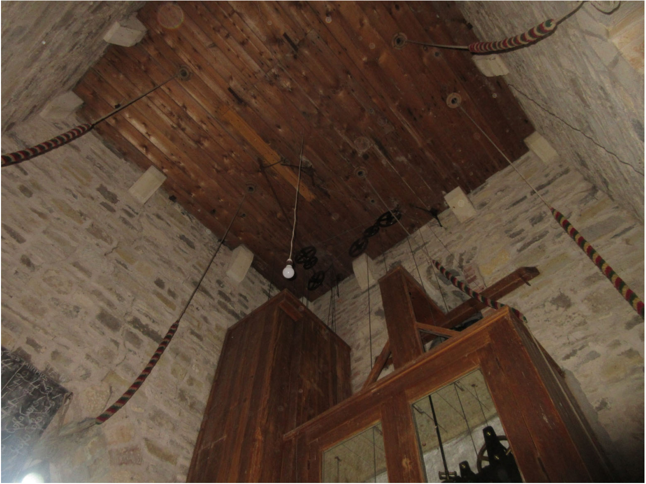
Above: The Ringing Chamber ceiling and clock.
