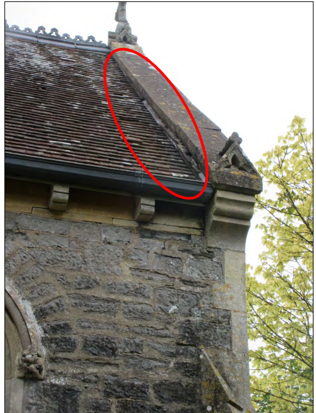
002 Detaching flashings on the chancel roof.
