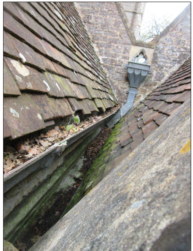
008 The narrow back gutter between the chancel and vestry roof.
