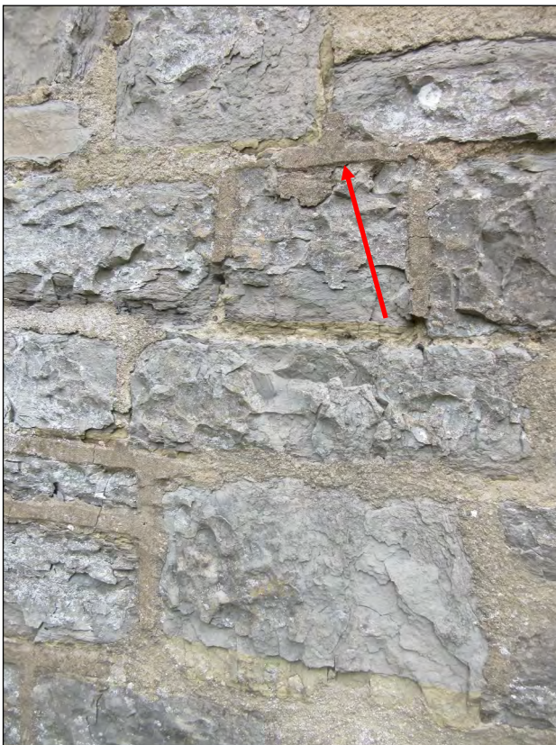
015 Typical cement pointing to the blue lias stone-work.
