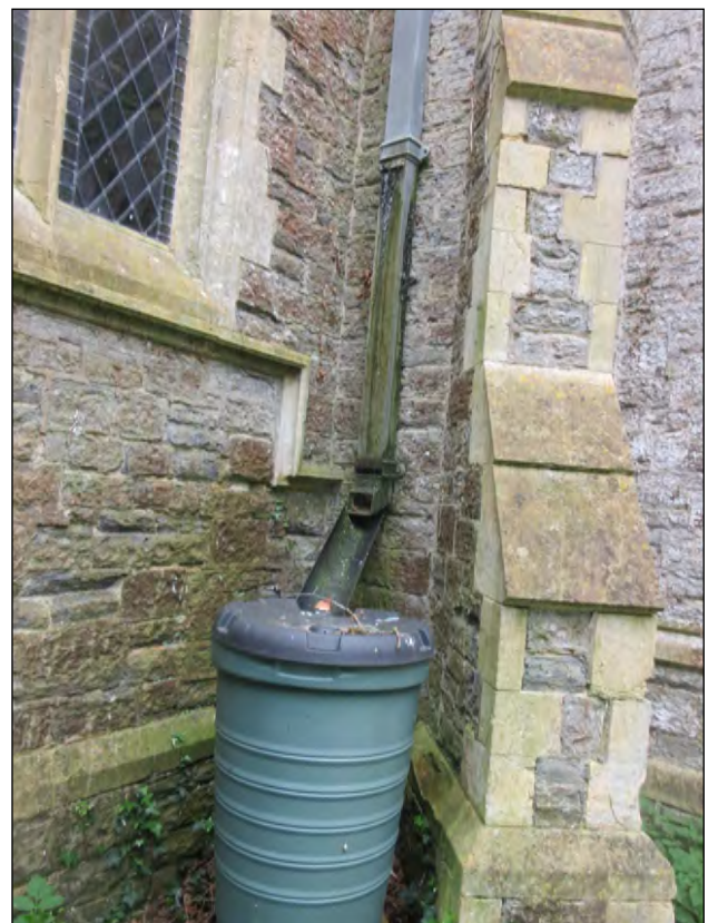
012 The water butt at the west end of the north aisle.
