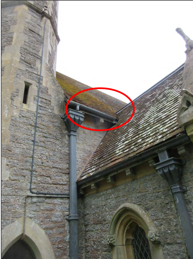
009 A section of uPVC guttering on the south side of the nave roof.
