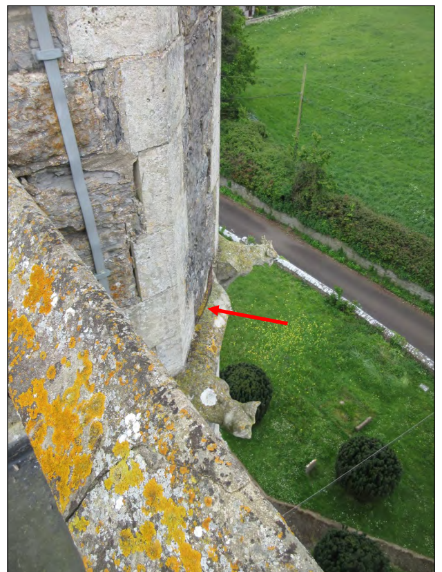
038 The iron band around the top of the vice turret.
