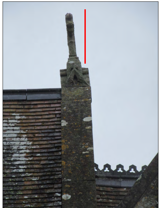
019 The backward leaning cross on the South Porch and the disturbed copings capping the wall below.
