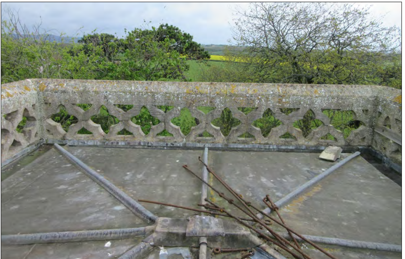
034 The tower roof.
