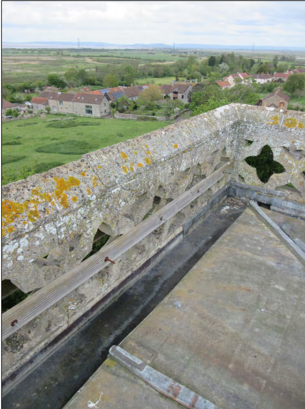
039 The north parapet of the tower roof,
