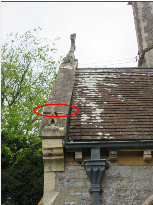
019 The backward leaning cross on the South Porch and the disturbed copings capping the wall below.
