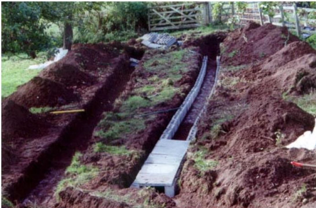
A trench arch being constructed. Fig 3
