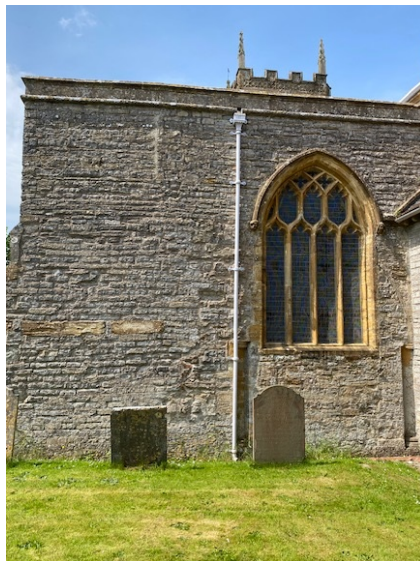
Photo 7 – East elevation of South Transept
