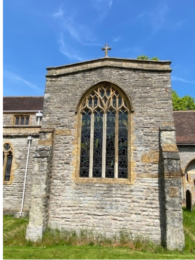
Photo 1 – South Elevation of South Transept
