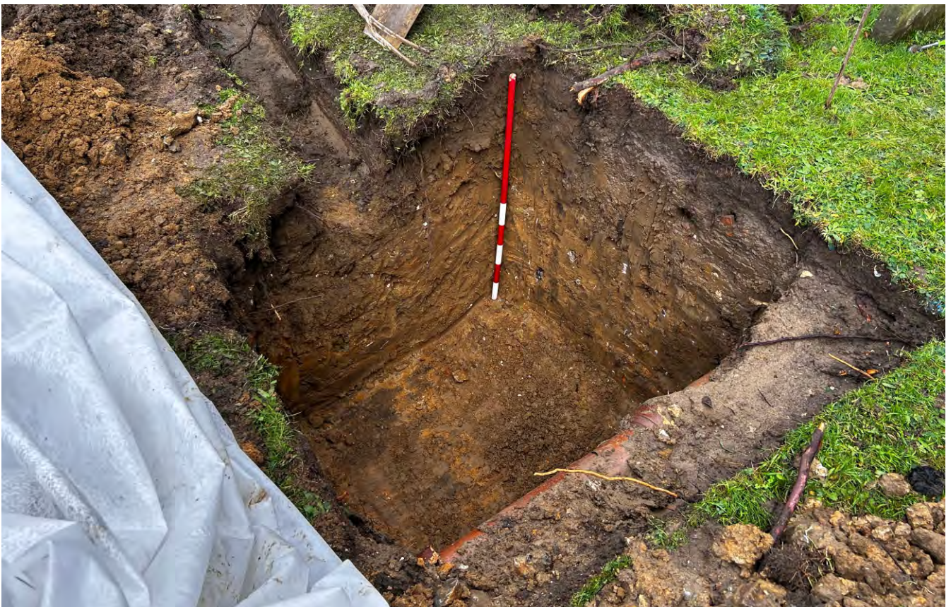
Plate 16. Detailed view looking into Soakaway 2 showing topsoil over disturbed churchyard soils sealing Superficial geology beneath with infilled graves extending beyond the excavation base.
