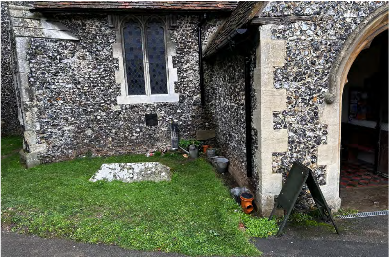
Plate 5. General view looking north along the proposed line of Trench 2 at the base of the South porch's western wall base from its junction with the south wall of the south aisle to the edge of the churchyard footpath (note: existing 'French drain' along the base of the porch's side wall).
