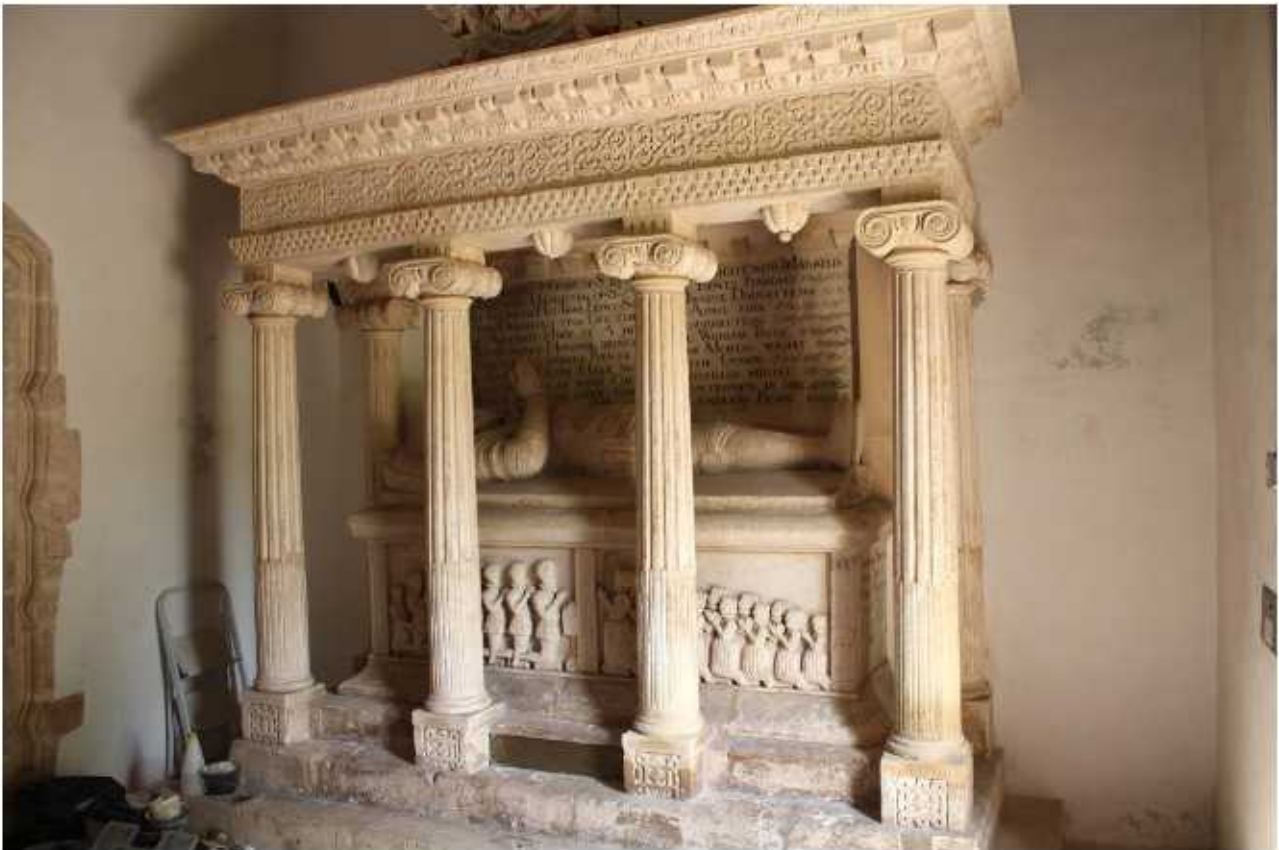
14. Monument after work was completed
