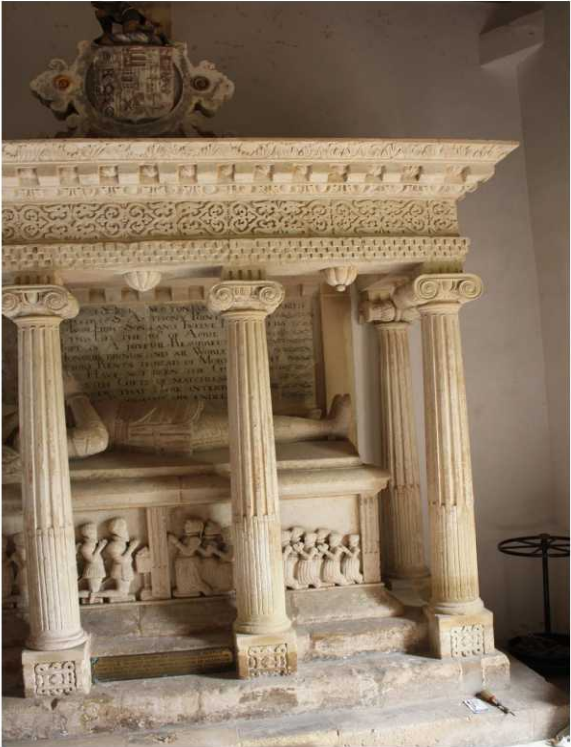
17. Southern end of monument after work
