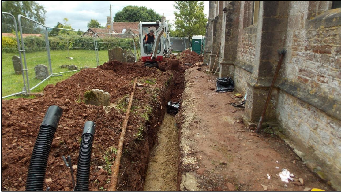
Figure 7. General view of removed path and service trench: facing E.
