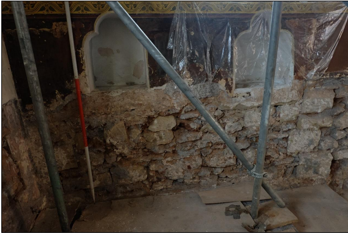
Figure 14. Chancel wall, E end: facing S, 1.5m scale.
