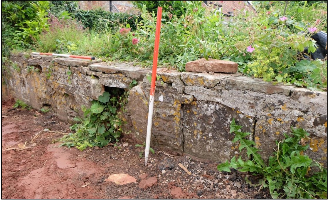
Figure 10. East gateway to South entrance wall: facing SE, 1m scale.
