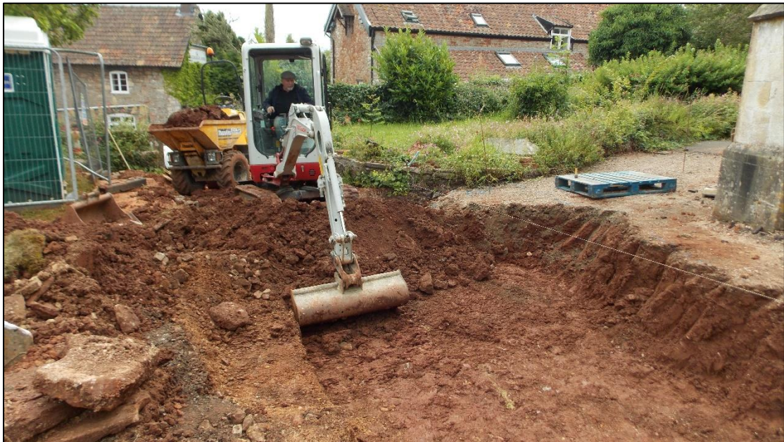
Figure 8. Pathway reduction in progress at east end of site: facing E.
