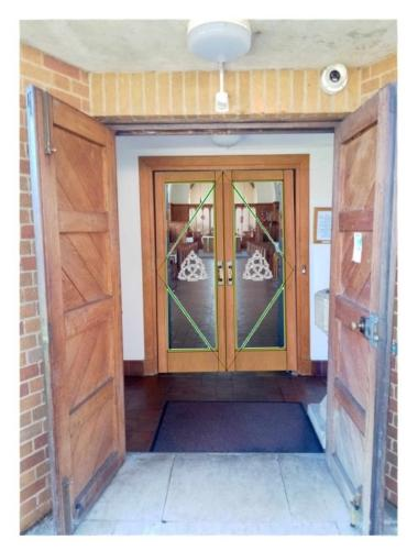
The replacement doors will use the existing handles which will be transferred across from the old doors. The new doors will be on new both-way swing hinges which will be lighter to use than the existing ones. The doors will be lighter in weight and will push open more easily and freely than the existing doors thus making them much easier to use, and more accessible for wheelchair users.
