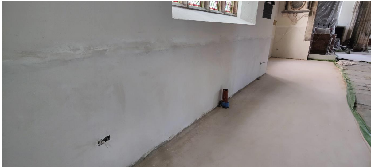
North aisle plaster repairs. Drying before painting.
