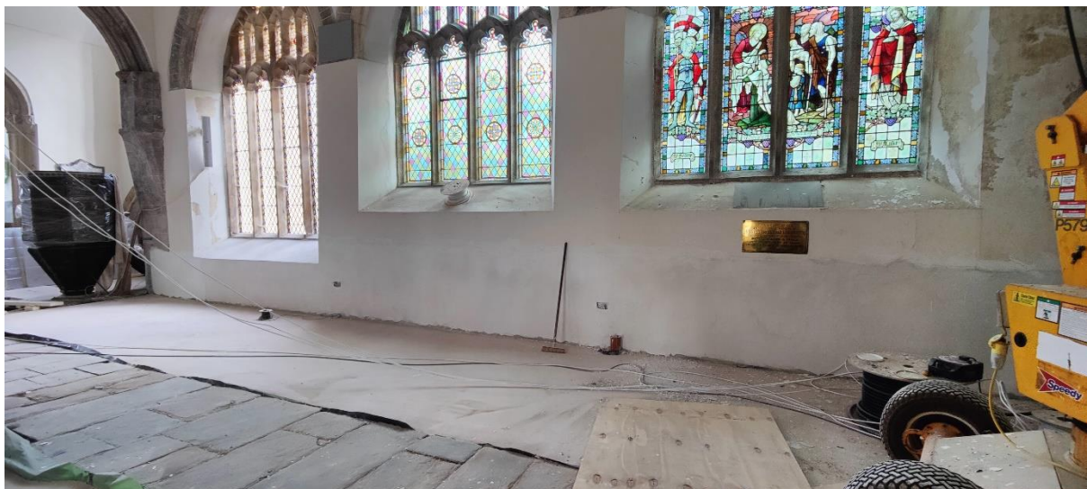
South aisle plaster repairs. Drying before painting.
