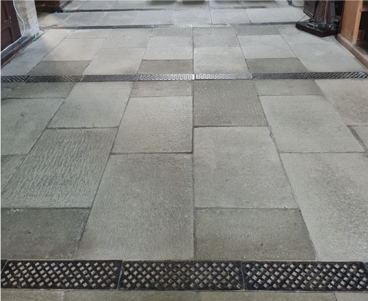
Typical finned pipe, gridded floor trenches
