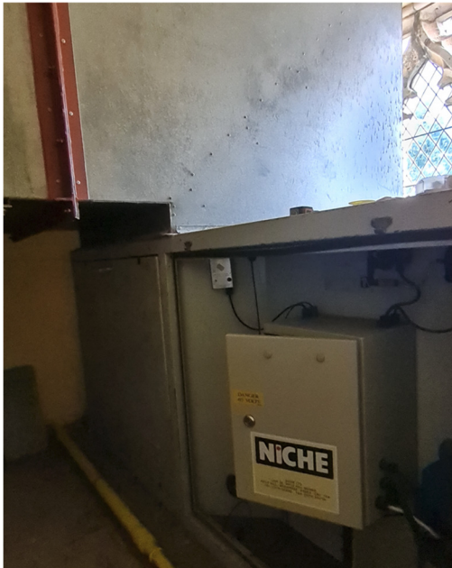
Existing Warm Air Heater Installation
