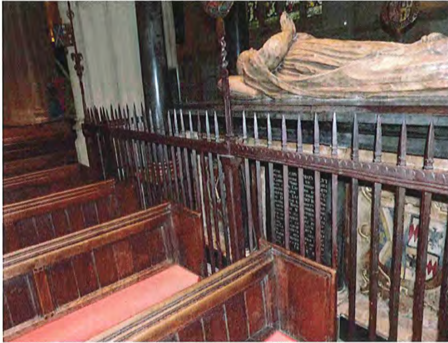
Fig 33: south side railings
