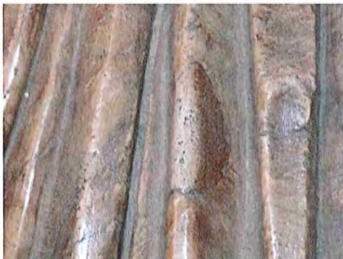
Fig 22: detail of repairs to effigy
