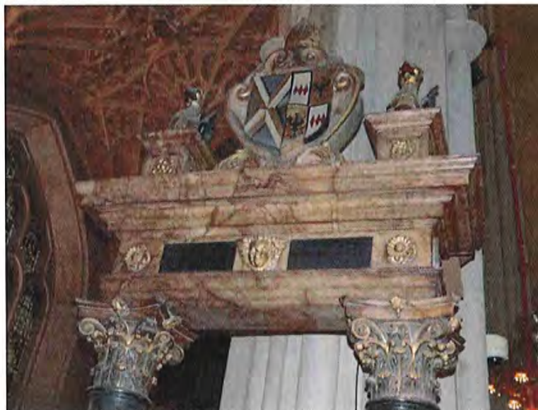
Fig 30: upper section of east entablature
