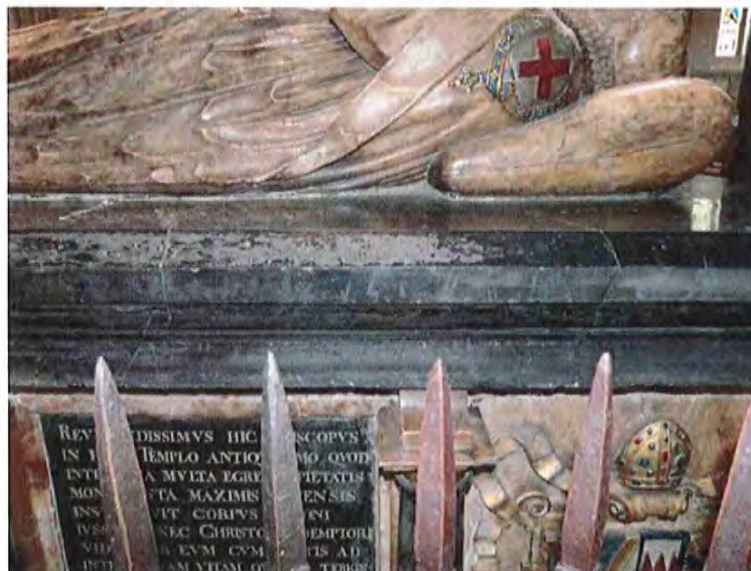
Fig 25: faults running across the slab
