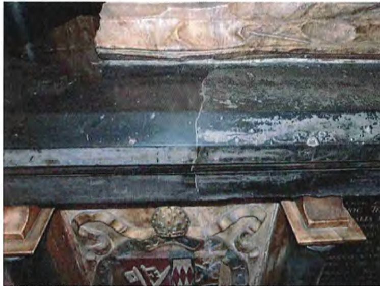
Fig 24: fault across slab with different surface effect on each side
