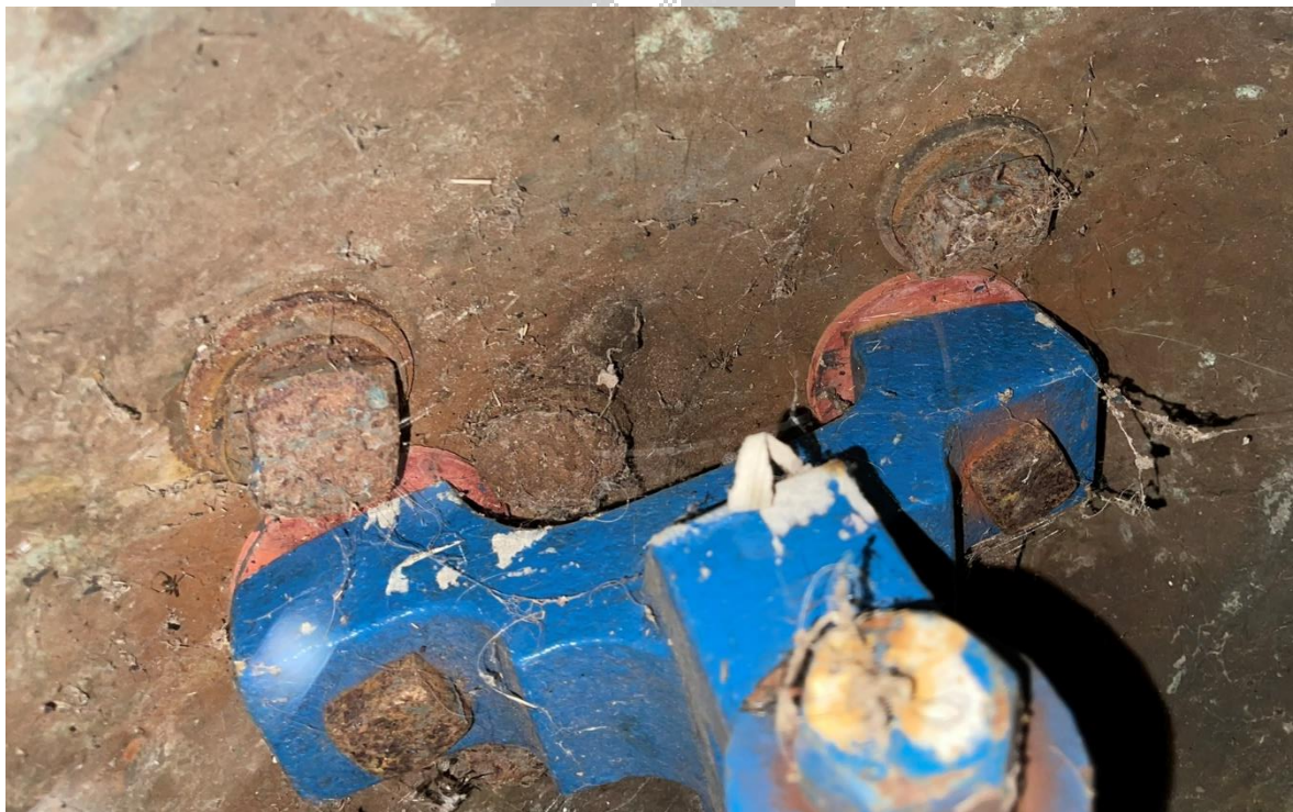
The crown staple of bell 6, showing the roots of the original cast-in crown staple.
