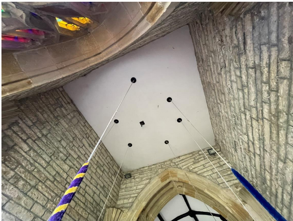
Looking up at the second floor – showing lack of trap door for the hoisting of bells and associated materials.
