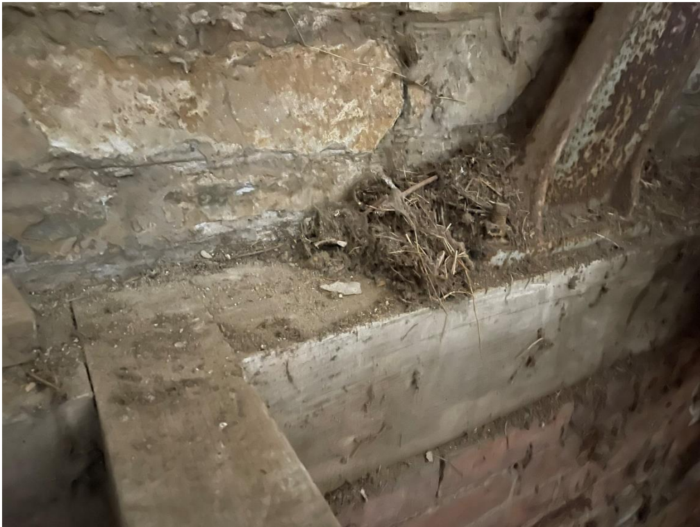
The accumulated dirt and nesting material, between the bellframe and the tower walls.
