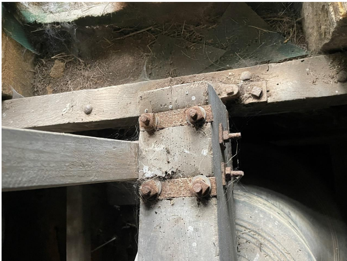
The poor state of the headstock of bell 6.
