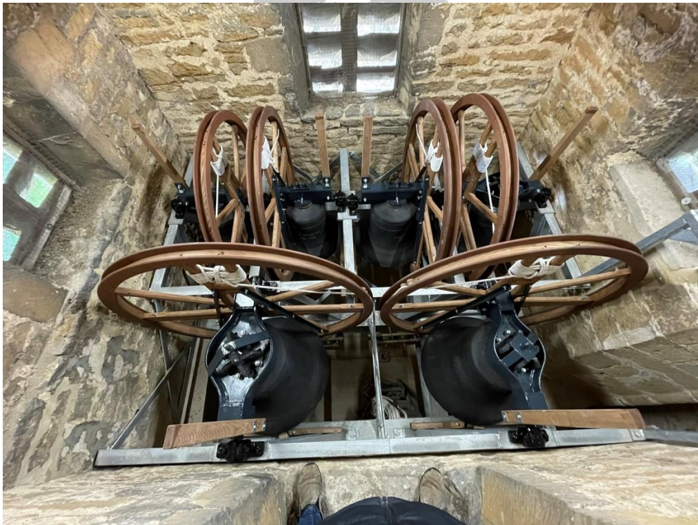
An example of a steel bellframe and modern fittings – Littleton Drew, Wiltshire, 2021.
