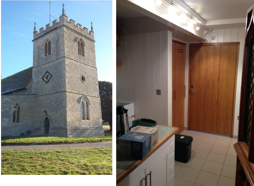
Figure 24: The Tower, with its internal ground-floor facilities.
