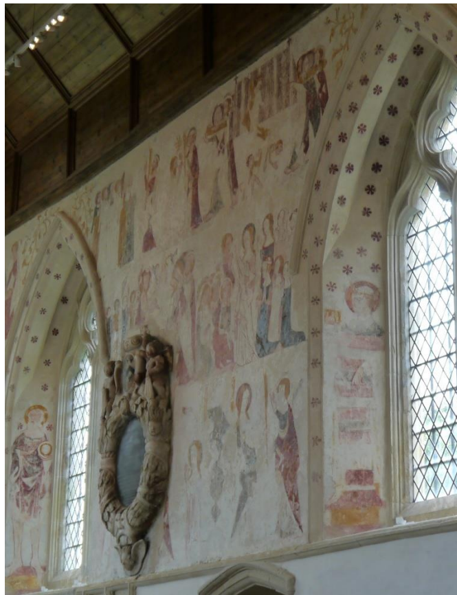
Figure 19: The wall paintings and Markham memorial on the south wall, between the two windows.
