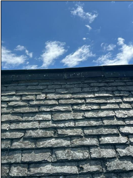
Ridge over chancel pointed
