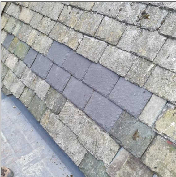
North pitch of chancel. Patch repair in new blue Westmoreland.
