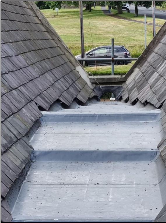
Looking West, Nave on left and North Aisle on right.
