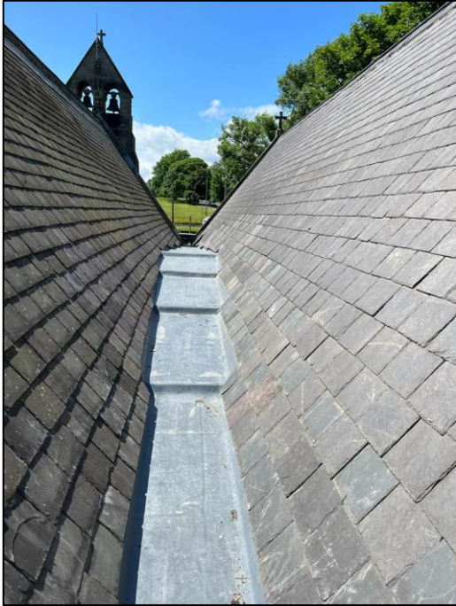
Central gutter cleaned of debris
