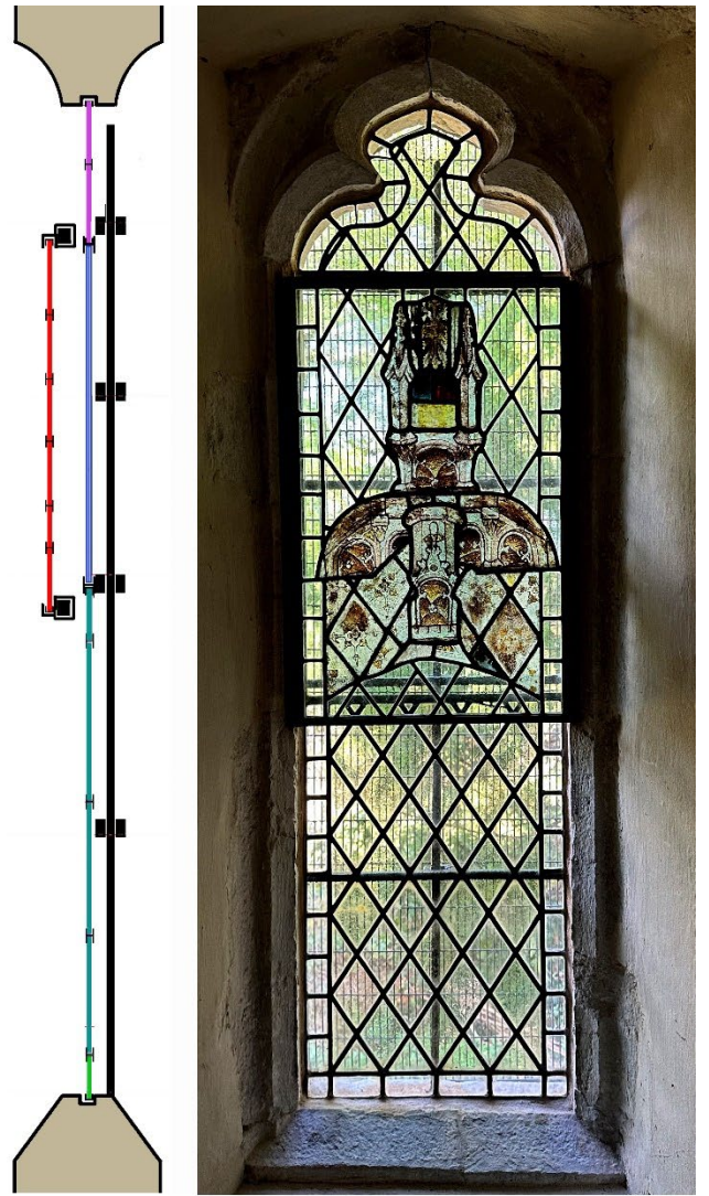
After conservation, showing new glazing arrangement
