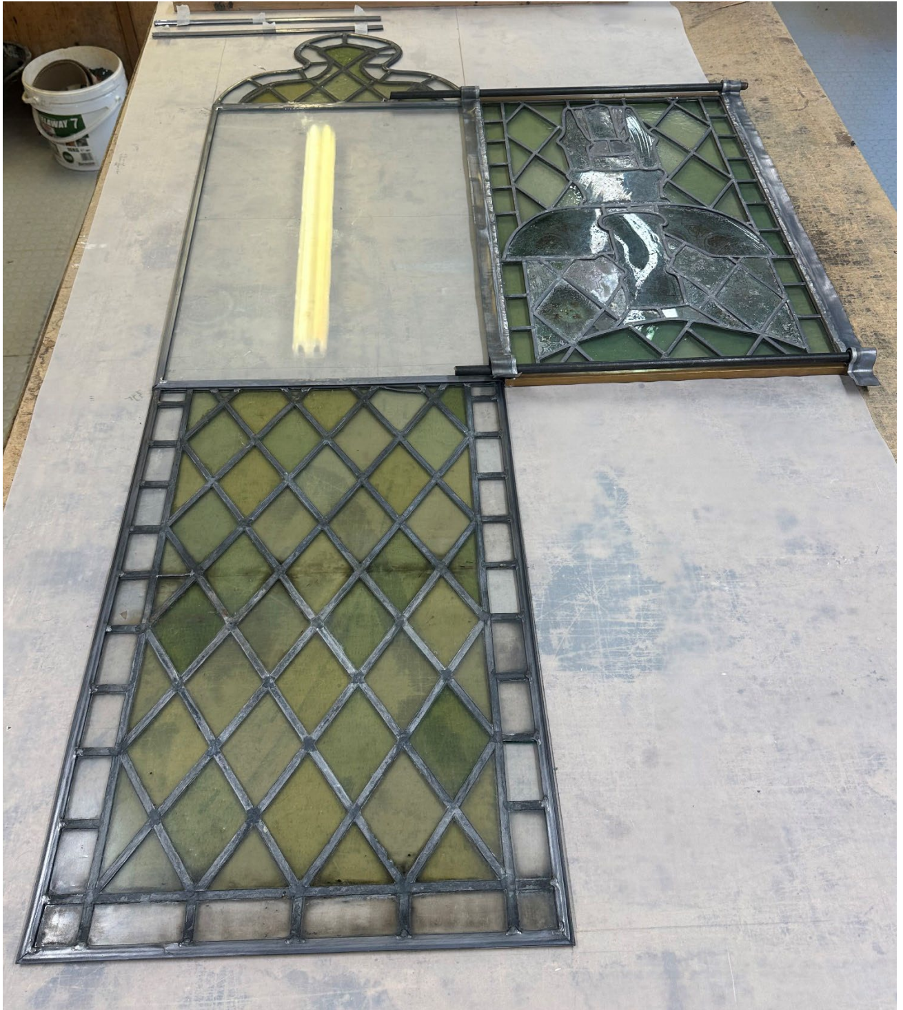
Above: the outer layer of glazing, with 19 th century diamond quarries in head and bottom panel, and a new laminate sheet of glass in the middle; the inner layer of glazing containing the medieval stained glass is now framed with a bronze U-channel and suspended with steel hoops on bronze bars set into the jambs. A strip of lead flashing prevents light creeping around the edges of the frame.
