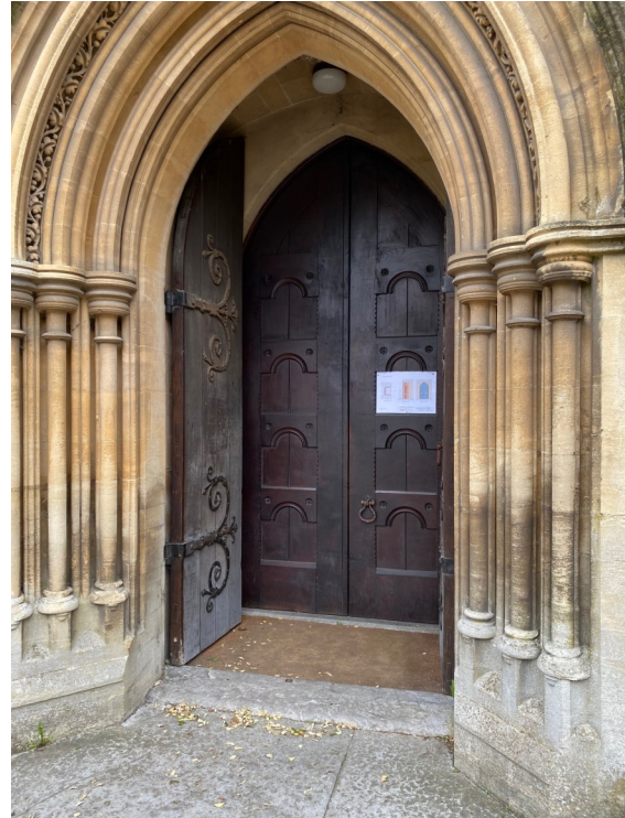
The internal doors viewed from outside.
