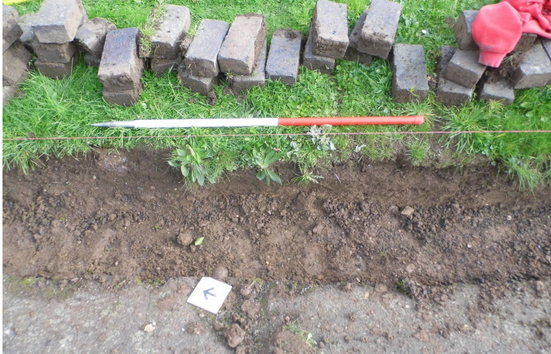
Figure 3: Section of brick removal from path looking north-east
