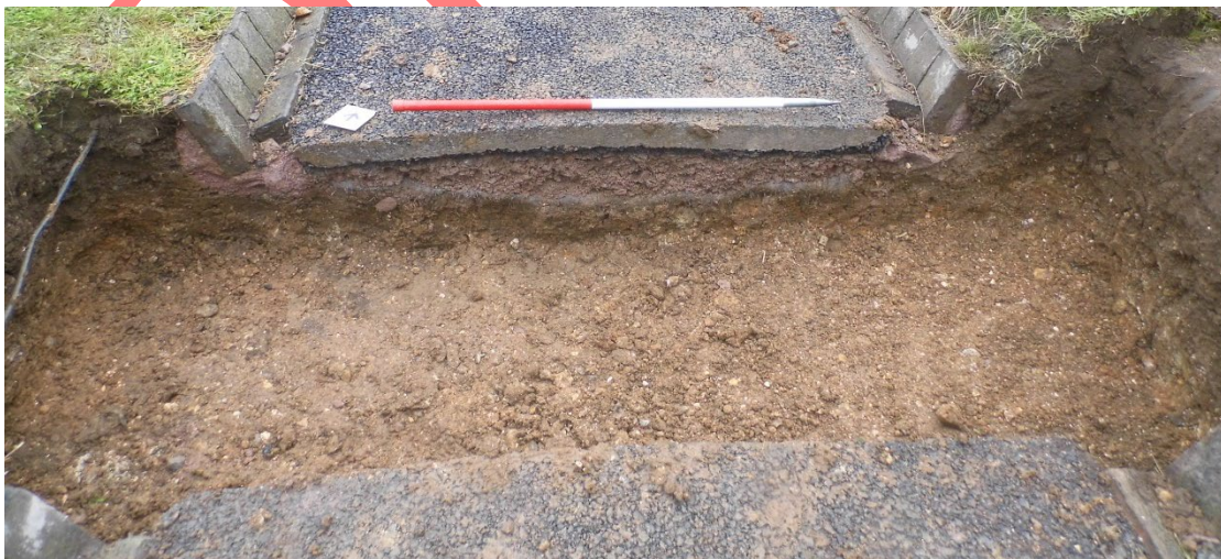
Figure 5: Excavated section through tarmac path looking north-west.
