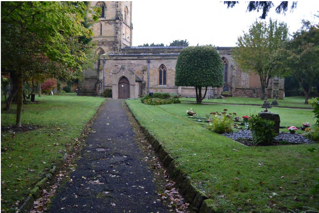
1 All Saints Church and path prior to excavation works
