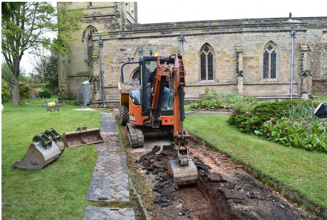
5 Excavation of the drainage trench
