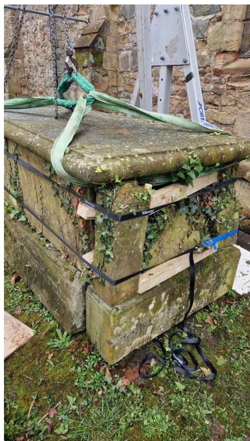
Plate 4: here we can see the east end of the tomb and the timber shoring with ratchet straps securing the stone panels. This method of shoring was also carried out to the west end also.
