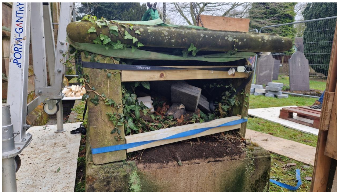
Plate 4: here we can see the east end of the tomb and the timber shoring with ratchet straps securing the stone panels. This method of shoring was also carried out to the west end also.
