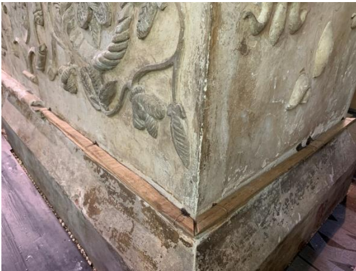
Plate 6: The lath fixed in place.
