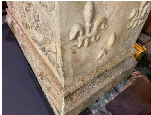
Plate 7: The backing coat for the moulding.
