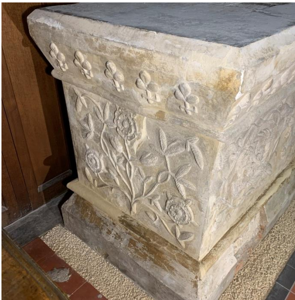
Plate 9: The west face after mortar repairs and reinstating moulding.
