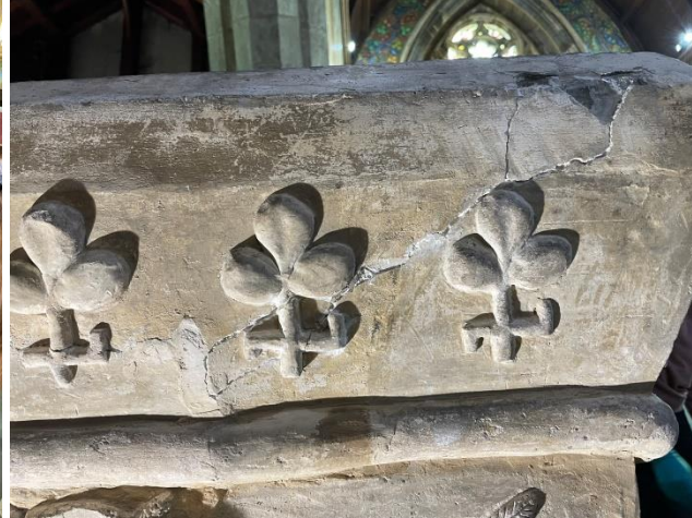
Plate 2 (left): The south face during consolidation
