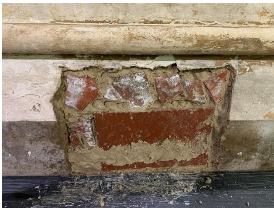
Plate 11: Building up the backing coats.
