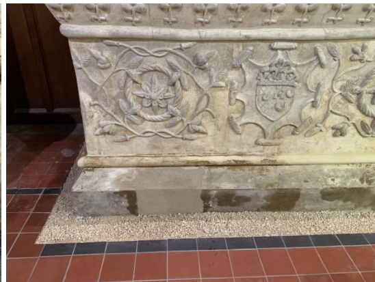
Plate 12: The top coat applied.
