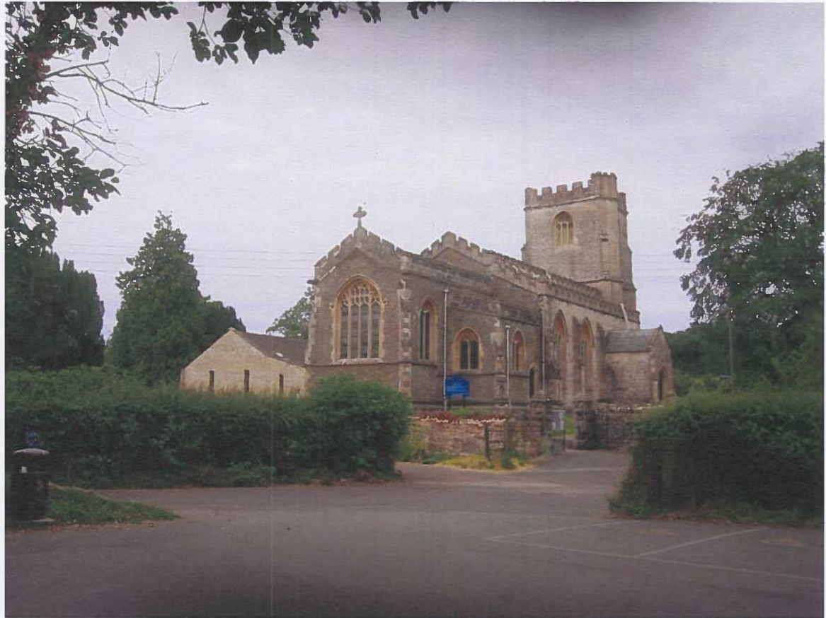
View from north east within existing carpark
