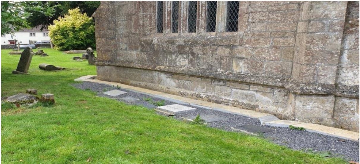
Figure 22: Repaired Ground Gullies
