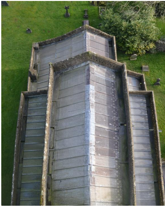
Figure 8: View from church tower showing Chancel (top of photograph), Nave and aisle roofs with stone parapets surrounding
