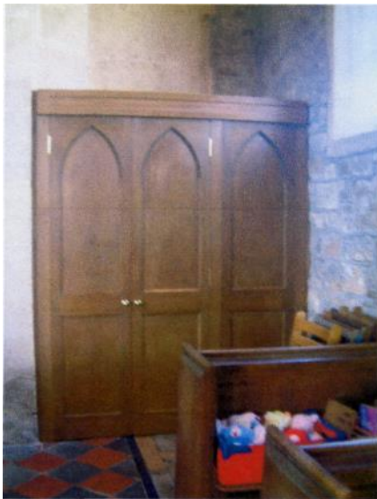
Figure 14: Cupboard N Aisle – removed in 2018 for installation of toilet facility. The adjacent window can be seen towards the top right of the photograph.
