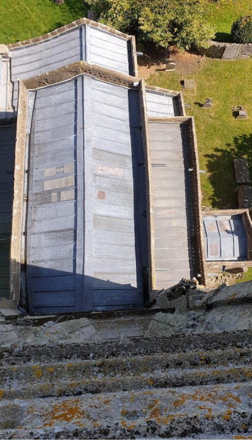
Figure 21: The lead roofs from the tower.
