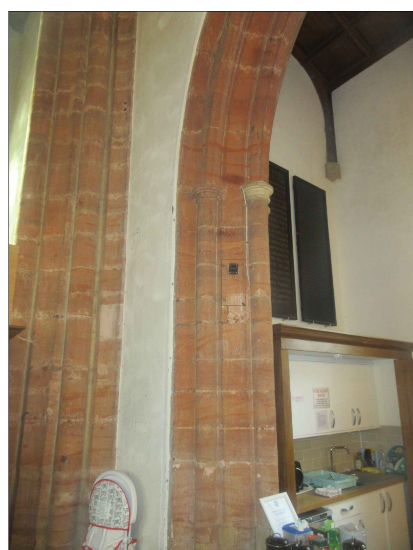
Speaker position No 1 West end of north arcade (Existing position)
