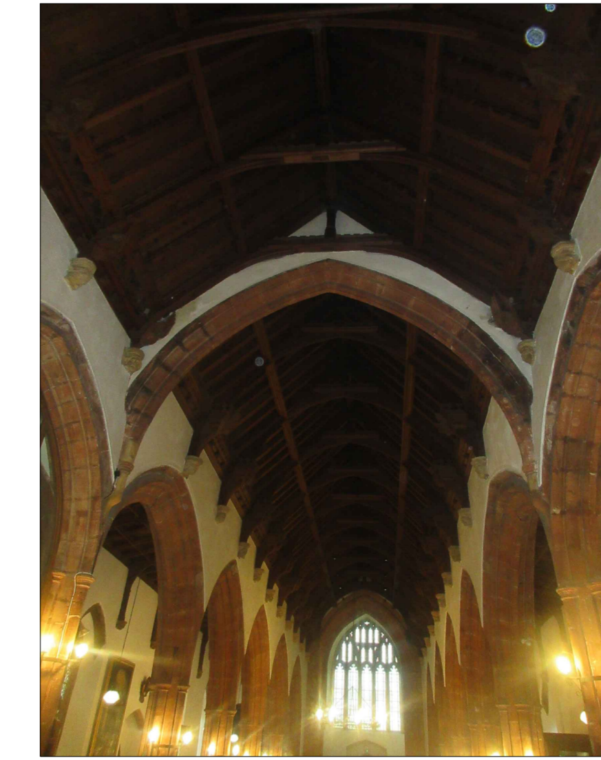
View of the nave from the chancel.
