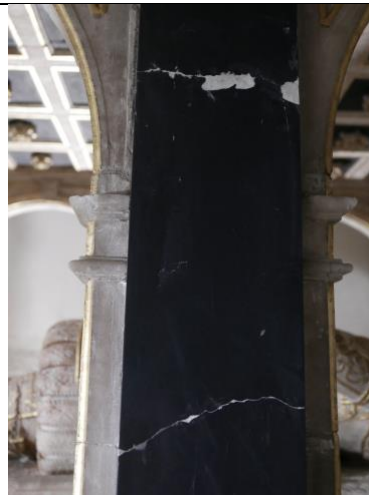
Fig. 34: plaster repairs on the column
