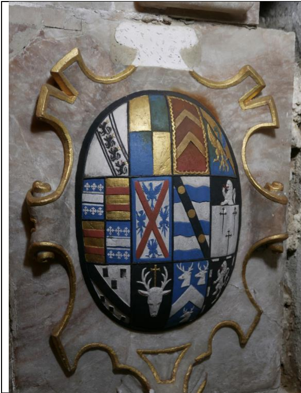
Fig. 43: detached volute above the heraldic shield
