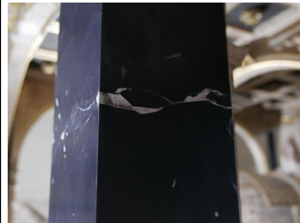
Fig. 33: plaster and Flügger fills on the marble columns
