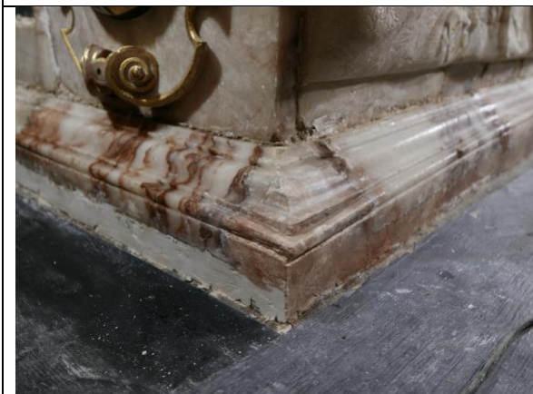
Fig. 29: reconstructed missing corner and the lowest section of alabaster (by the floor); photograph taken during retouching works
