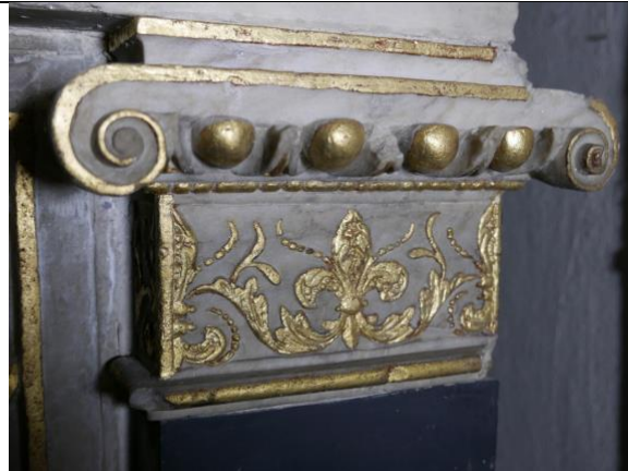
Fig. 21: capital of the column before wet cleaning
