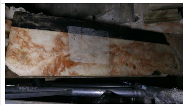
Fig. 11: square section of alabaster before wet cleaning; noticeable difference between cleaned and non cleaned stone surface
