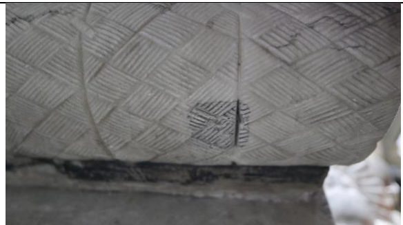
Fig. 54: another fixing hole repaired with plaster, presumably in 1956
