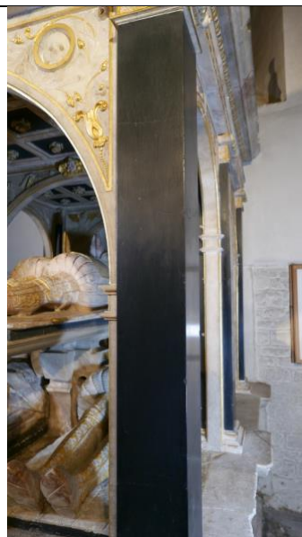
Fig. 36: the shaft after repairs and treatment with wax mixed with ivory black pigment
