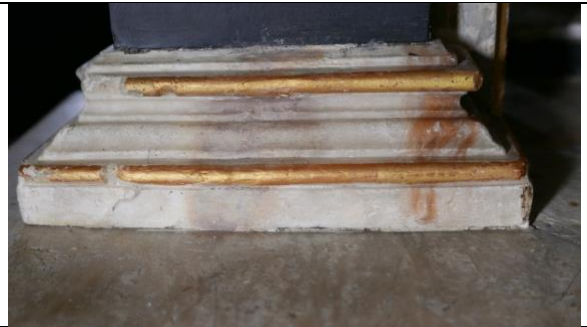
Fig. 32: the same section after repointing, reconstruction repairs and retouching
