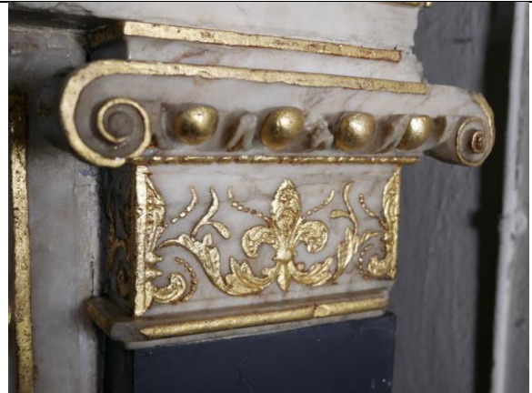
Fig. 22: warm colours of the stone and glow of gilding revealed after cleaning
