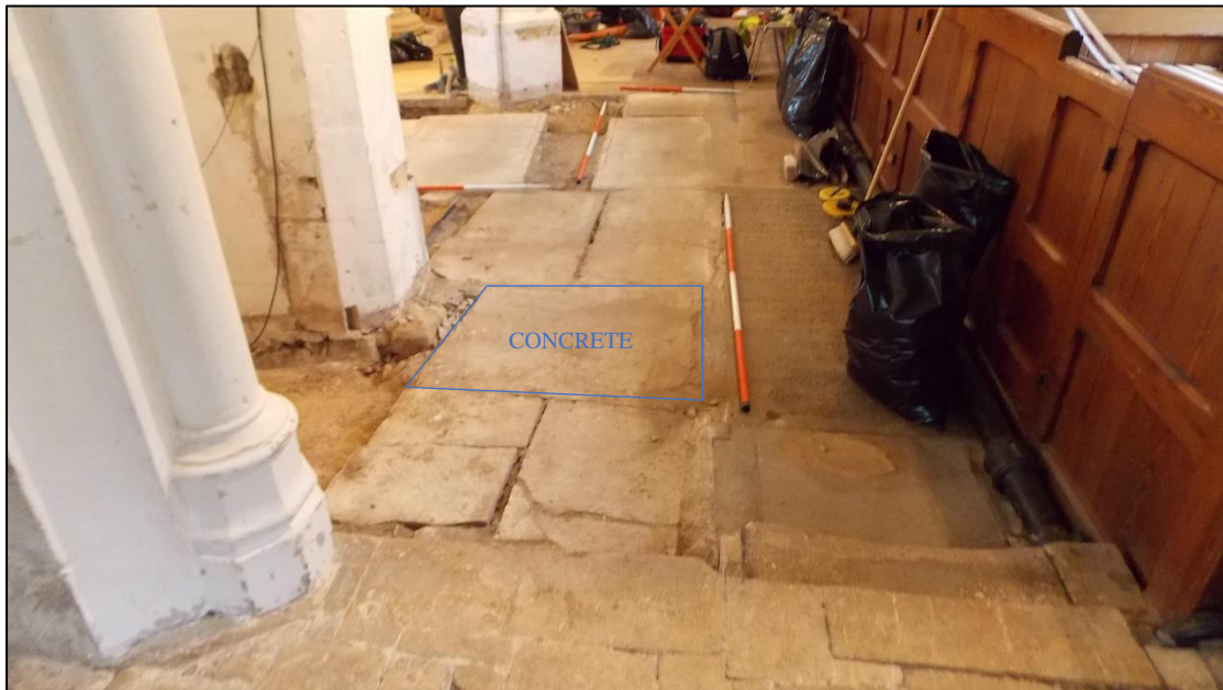
Figure 5. Remains of Bath Stone flooring & Concrete: facing W, 2m scale
