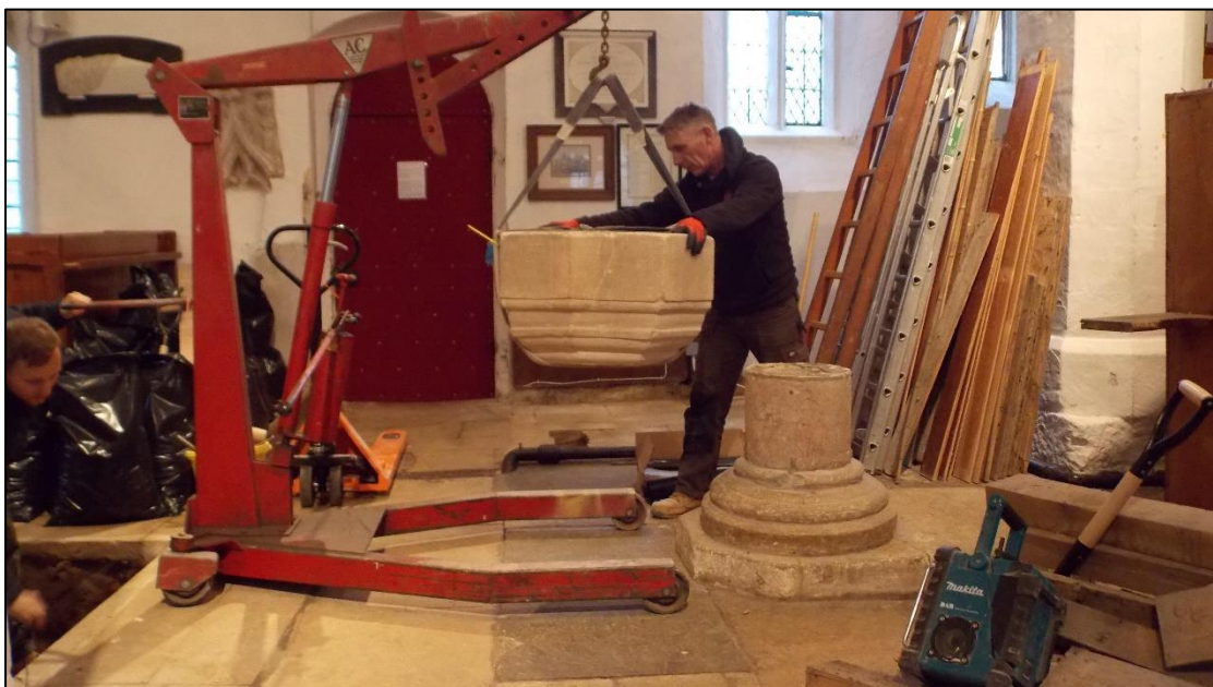
Figure 17. Removal of top section of font: facing S
