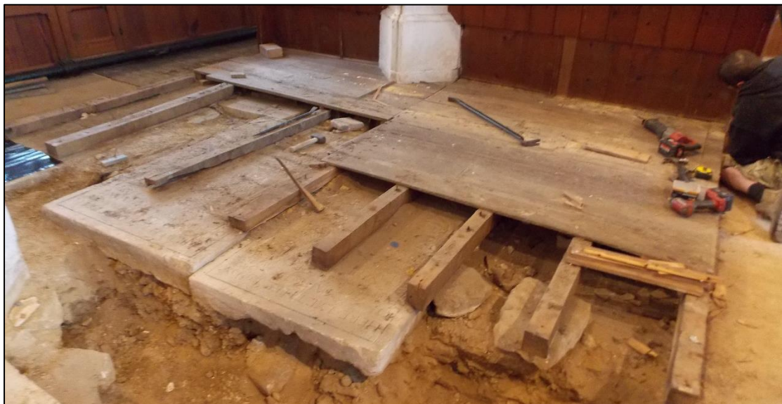
Figure 4. Timber joists resting on Ledger Stones: facing NE
