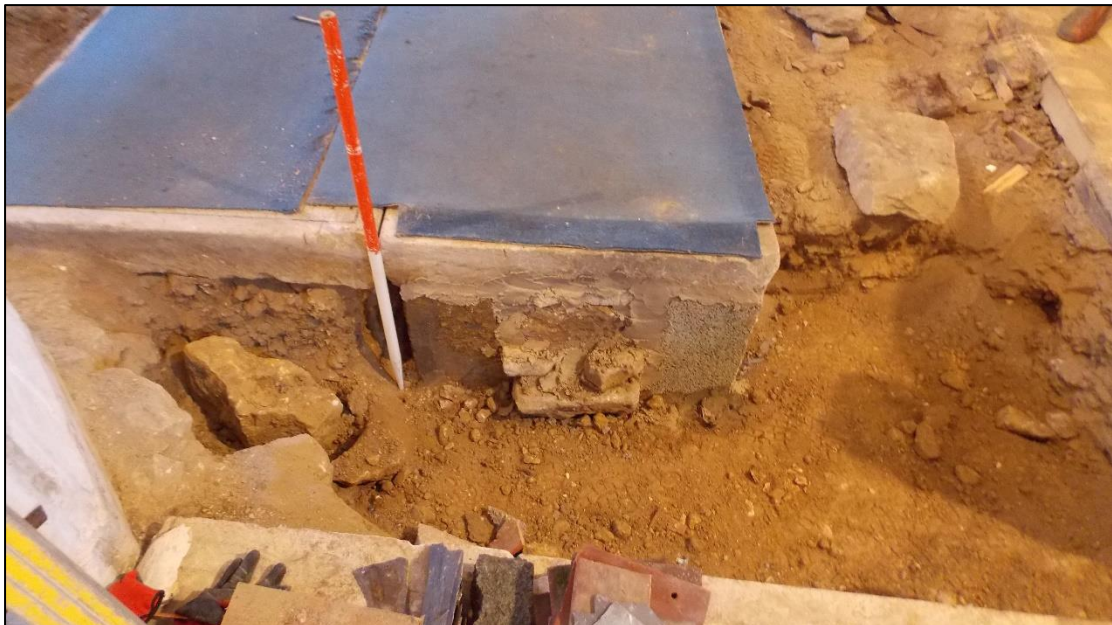
Figure 15. Supporting wall, W end of Ledger Stone: facing E, 1m scale
