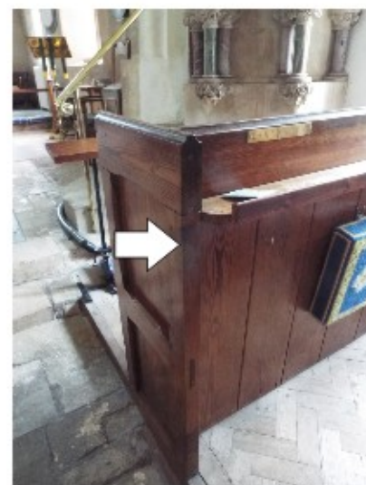
Benches (3) showing empty hinge rebates
