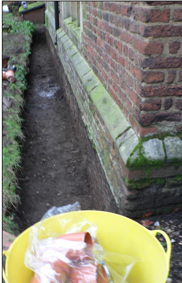
Trench from west
