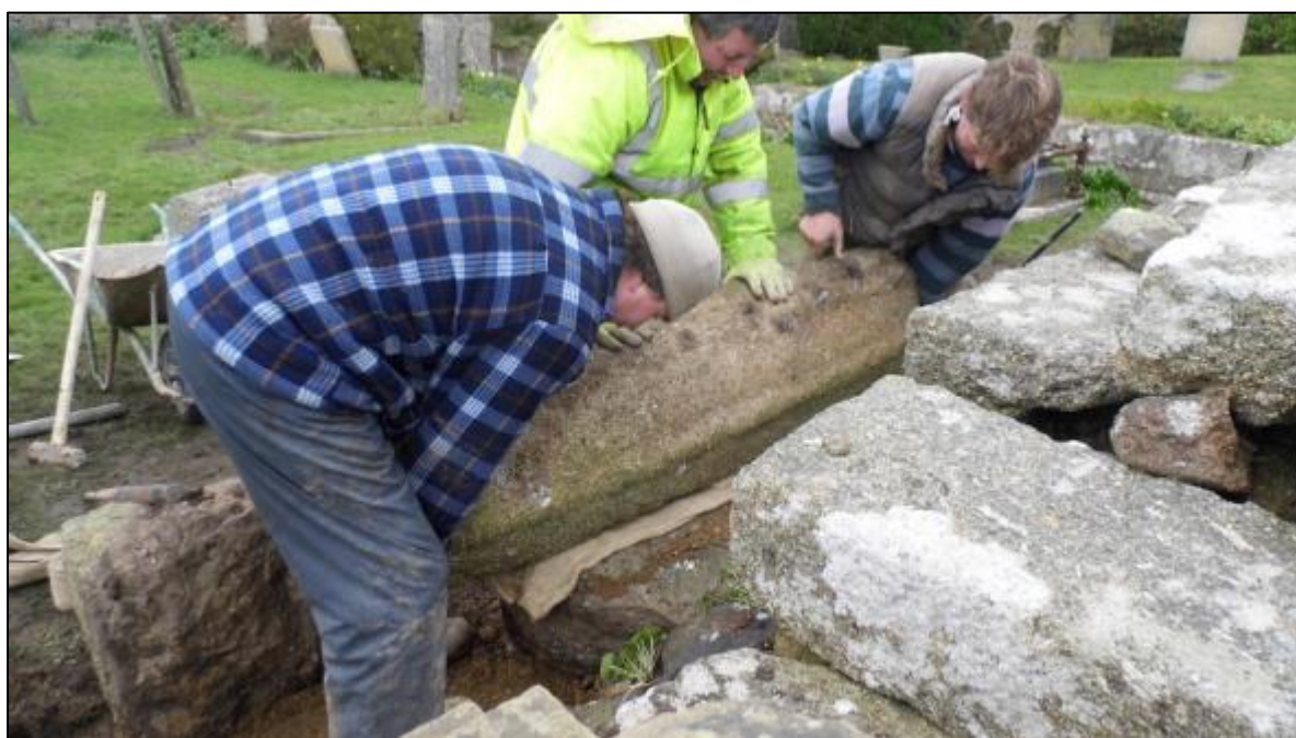
Fig 29 Conservation work in progress: the grave slab being moved aside (AGL).
