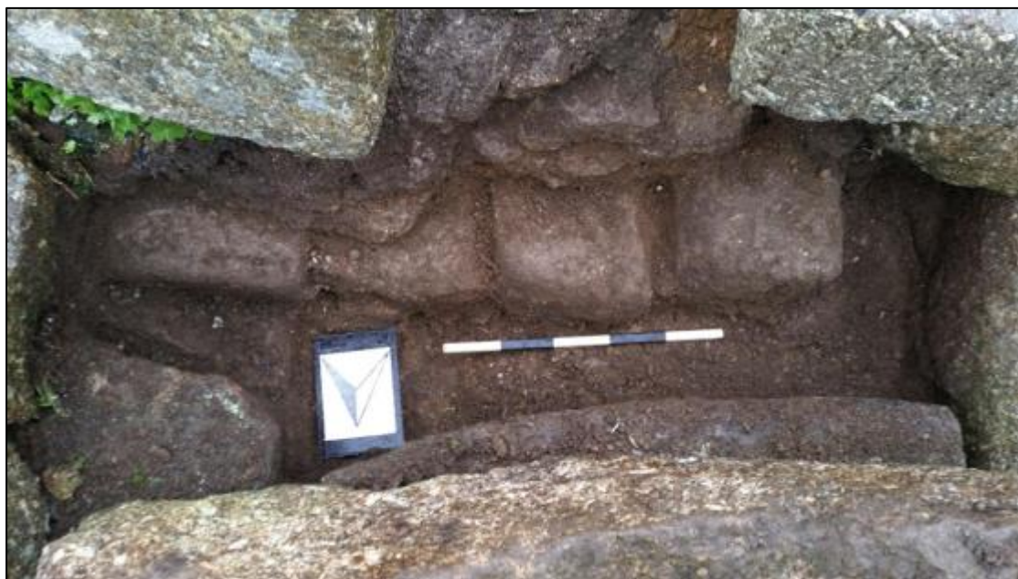
Fig 27 Wall or face of older step hidden within the nineteenth century 'shell', north-west corner (RS).
