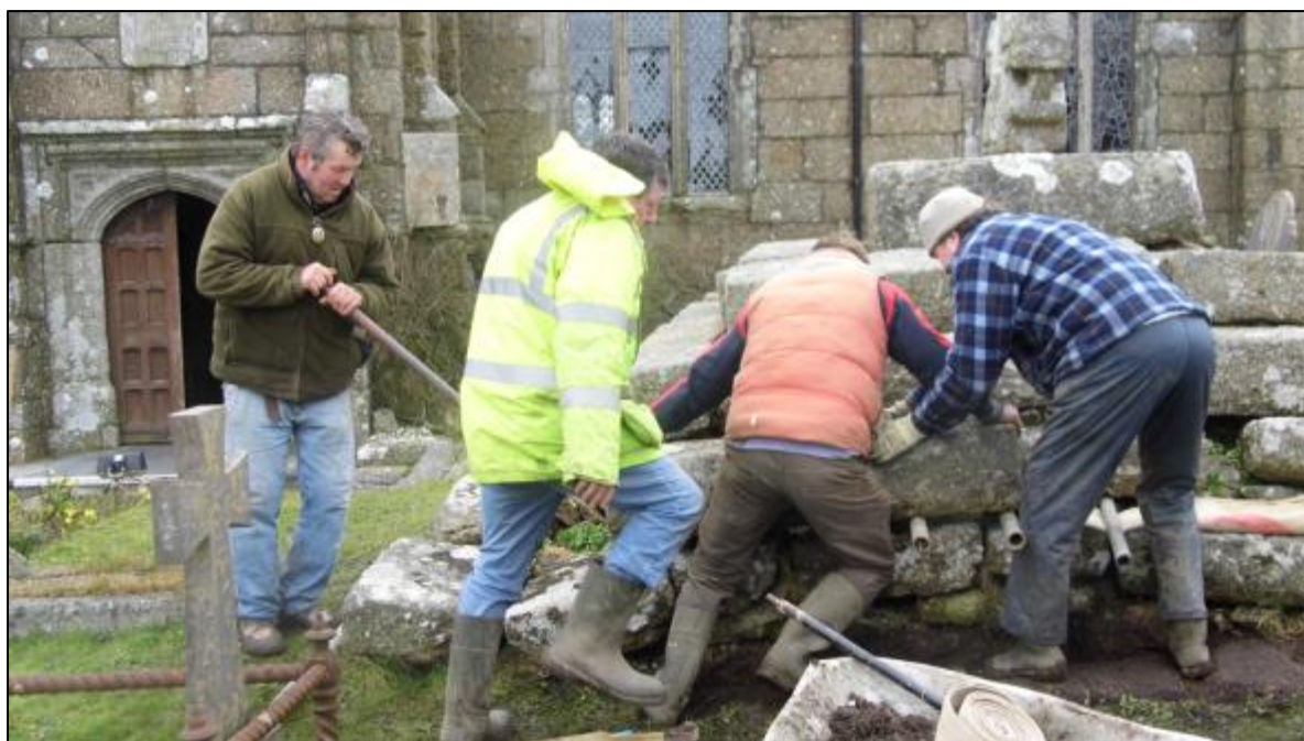
Fig 28 Conservation work begins on the south-west corner (AGL).
