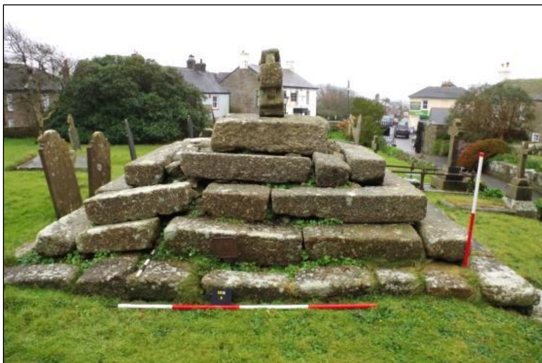
Fig 15 North elevation, showing slumping towards the east (left) (JG).
