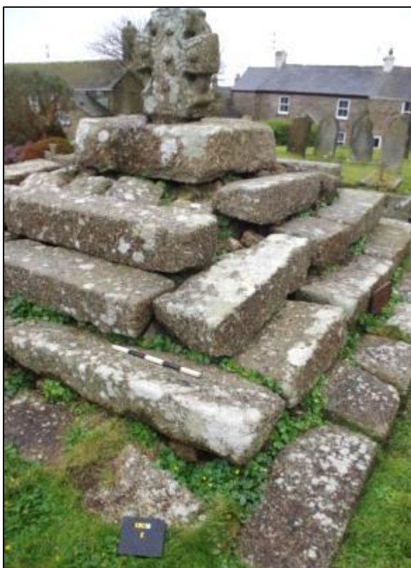
Fig 13 North east corner (JG).
