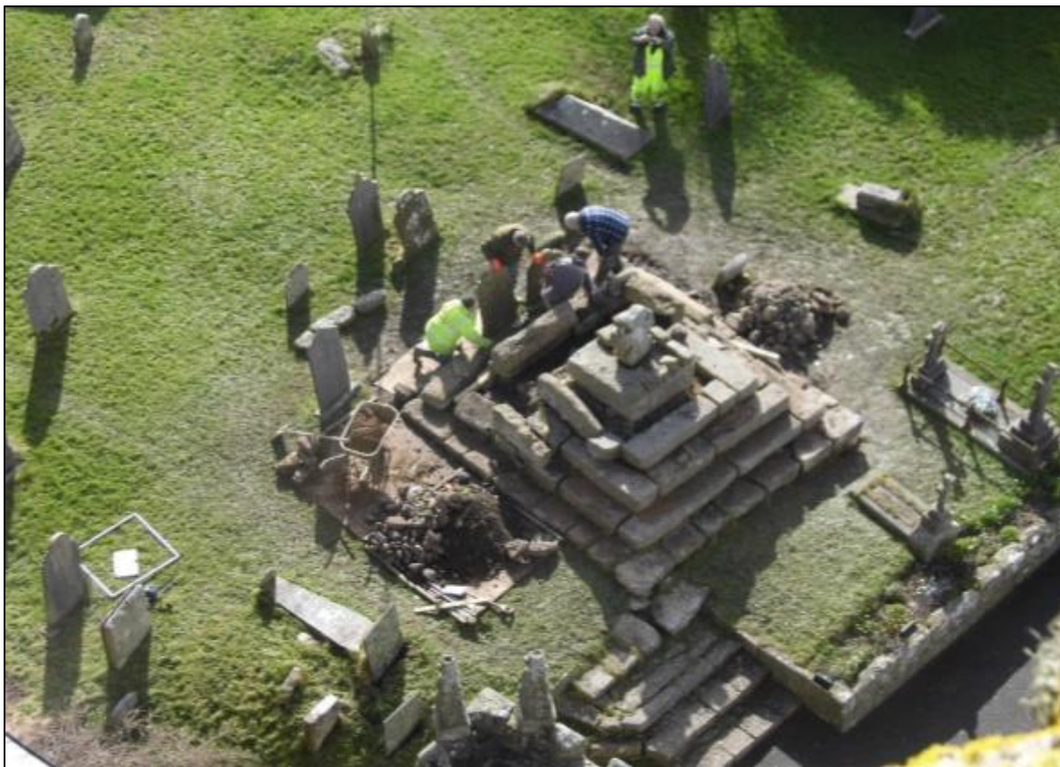
Fig 30 Conservation work in progress: view from the tower (AGL).
