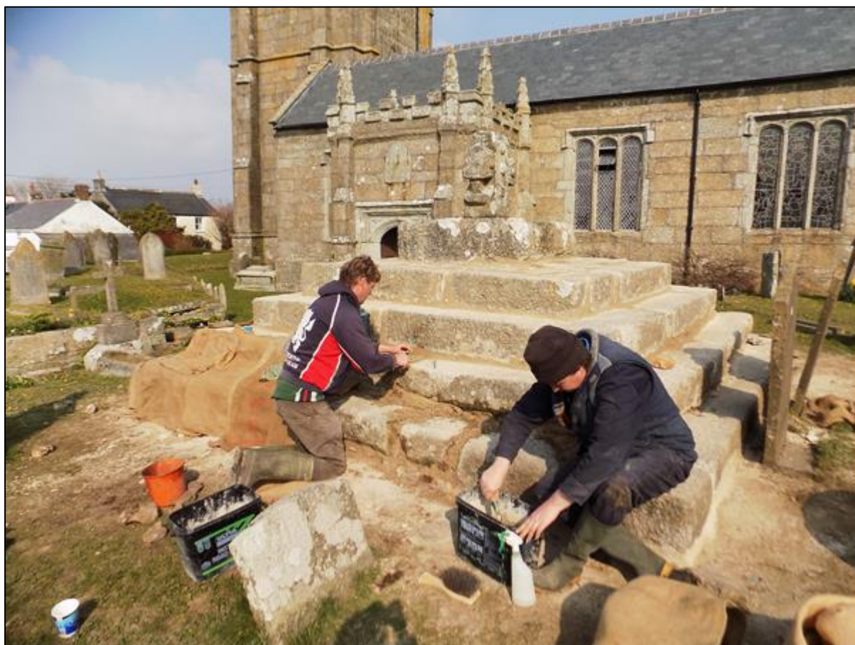
Fig 32 Conservation work in progress: deep pointing of the joints of the cross pedestal in a lime-based mortar (AGL, APJ).
