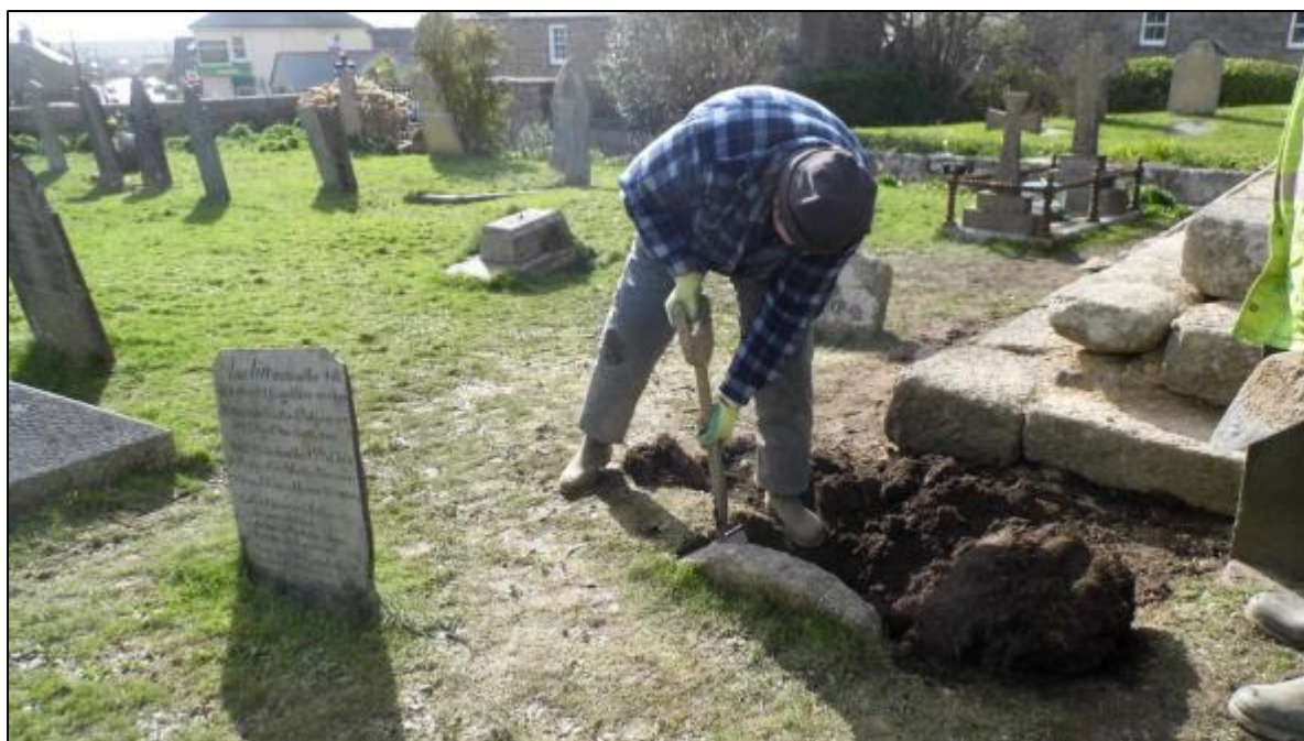
Fig 33 Conservation work in progress: raising an early headstone adjacent to the cross (AGL).
