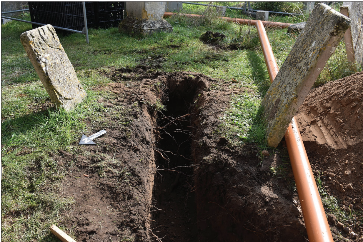
Plate 2: Drain trench through disturbed ground between two possibly relocated gravestones, looking south-east
