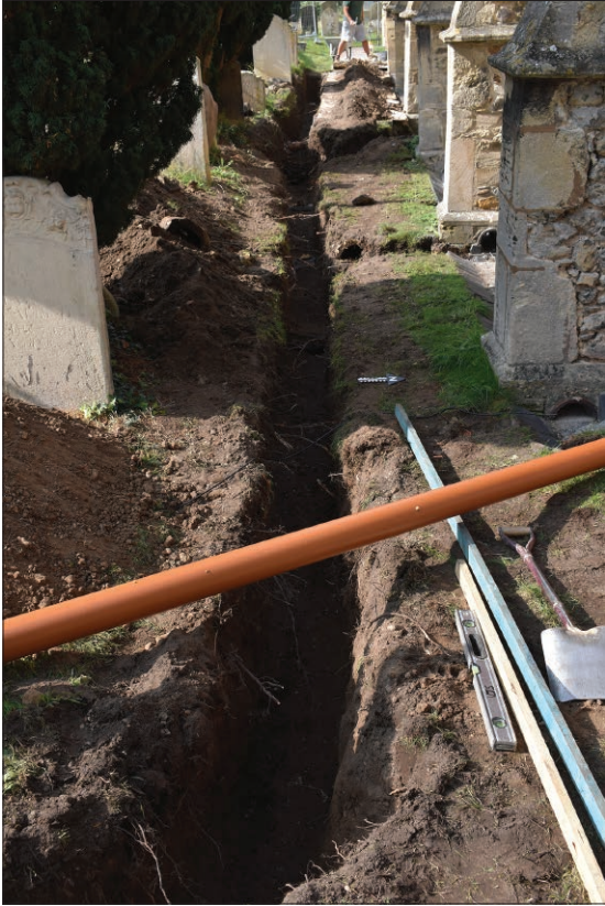
Plate 1: Drain trench through disturbed ground (18), looking west
