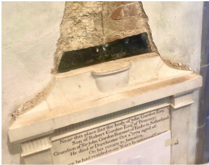
Figure 12 ~ Image of mantel, in situ, of retaining cramp location, front face, rear face, historic cracks to left and right shoulders.
