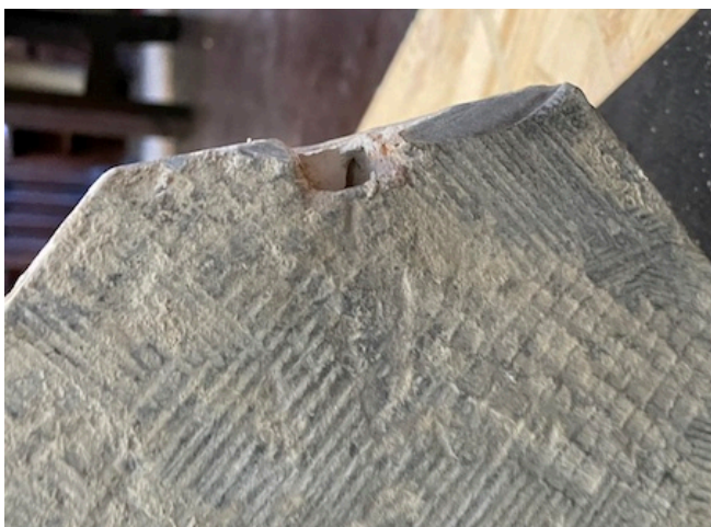
Figure 11 ~ Details or Urn and Ground. Lower left image illustrates retaining cramp location.
