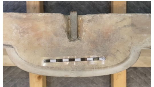
Figure 12 ~ Image of mantel, in situ, of retaining cramp location, front face, rear face, historic cracks to left and right shoulders.
