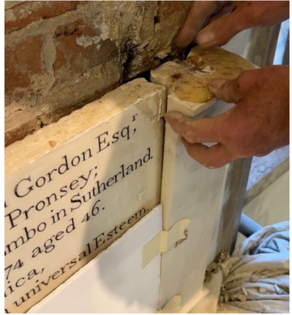
Figure 15 ~ Details of removal of pilasters and cramps.
