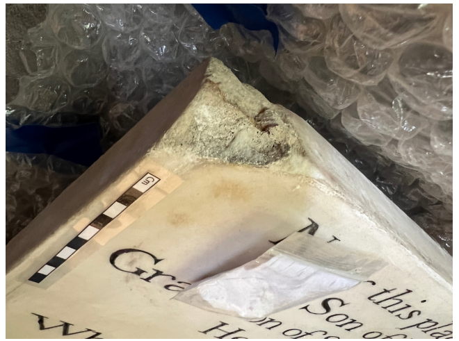
Figure 21 ~ Details of historic repairs to upper corners of inscription panel.
