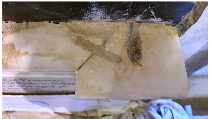
Figure 13 ~ Capitals flanking frieze in-situ, with details of: cramps to wall and to adjacent frieze element; front face; rear face; upper face; lower face.
