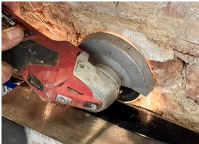
Figure 19 ~ Inscription panel. from top: in-situ; detail of retaining clamp; protections prior to cutting clamp; cutting clamp.
