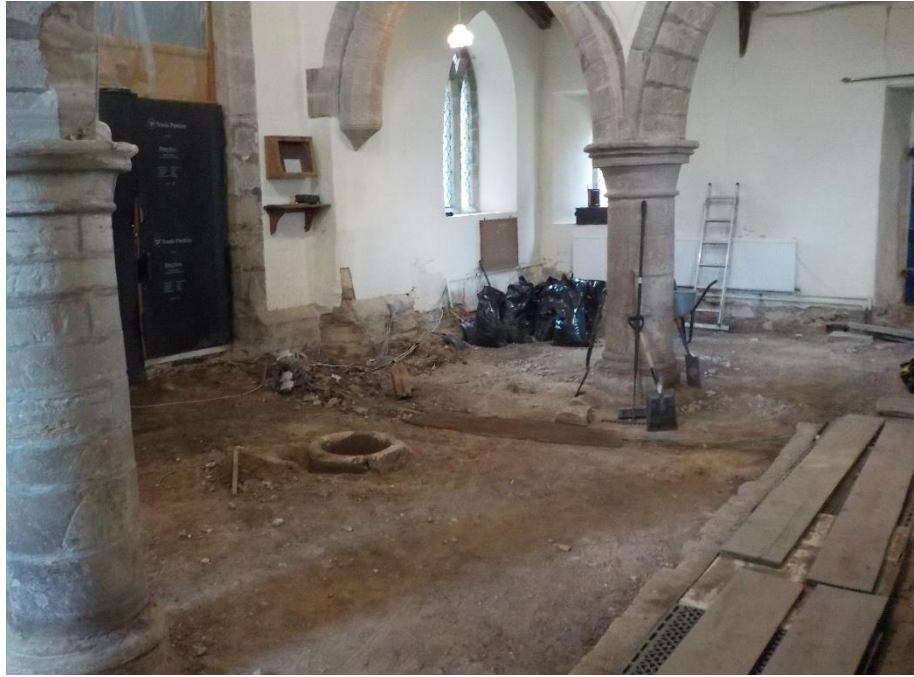
Plate 7. General view of area at formation level of excavation, facing north-west
