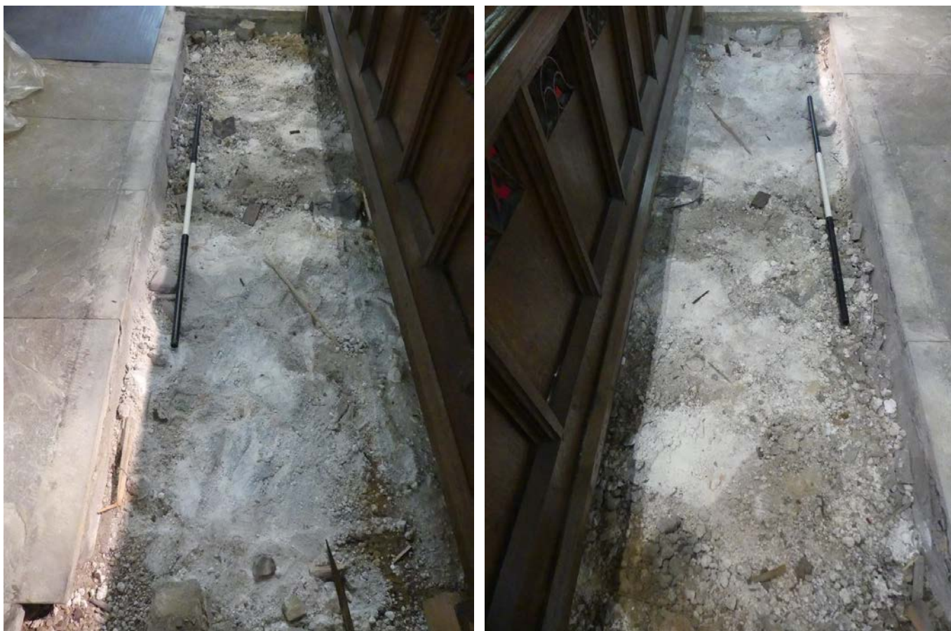
Plate 7 (left): Area 3a viewed from the north
