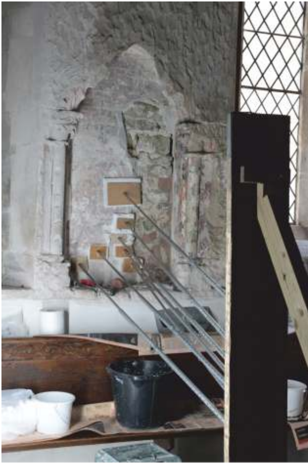
5 - Above - Securing detached plaster, 2023.
