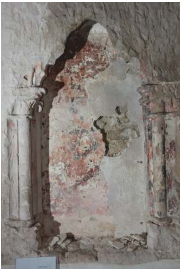
3 - Below - The detached plaster 2022.
