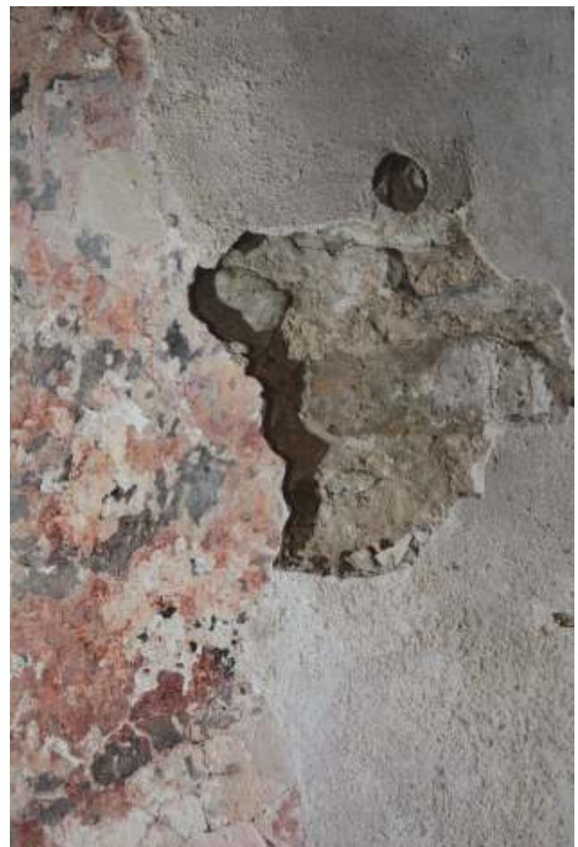
4 - Below - Detail from 3 showing the detached painted.
