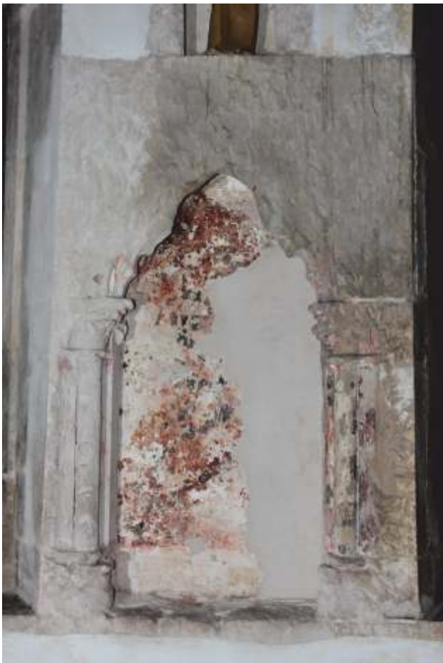
7 - Below - The niche following conservation and plaster repair, 2023.
