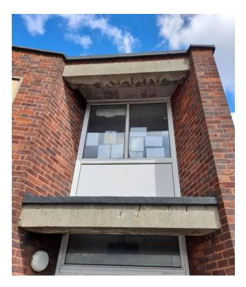
Loss of material of the concrete lintels has occurred on the building façade, leading to exposure of the reinforcing bars. These are made of steel and have begun to rust and expand, which will result in further concrete loss from the surface. The surface should be professionally repaired before damage becomes greater – contact your inspecting architect for advice.
