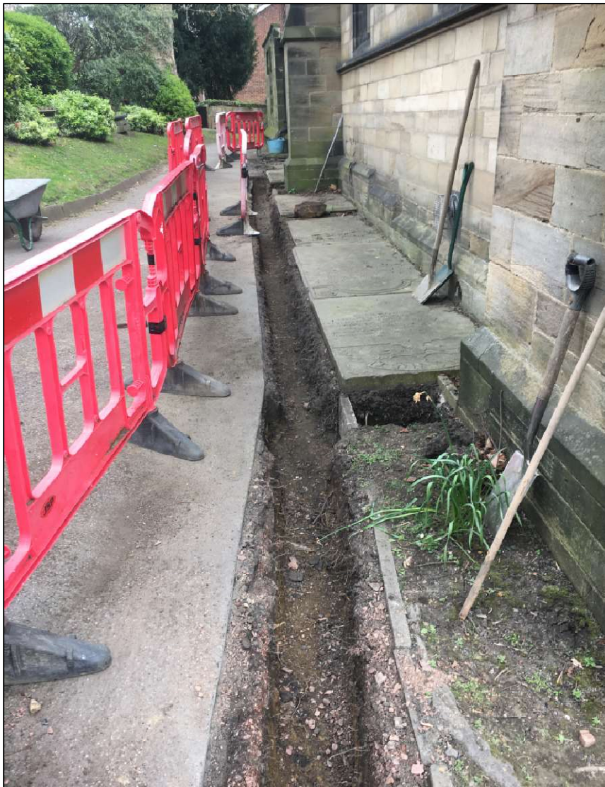
Plate 1. Drain run to north of church, looking east
