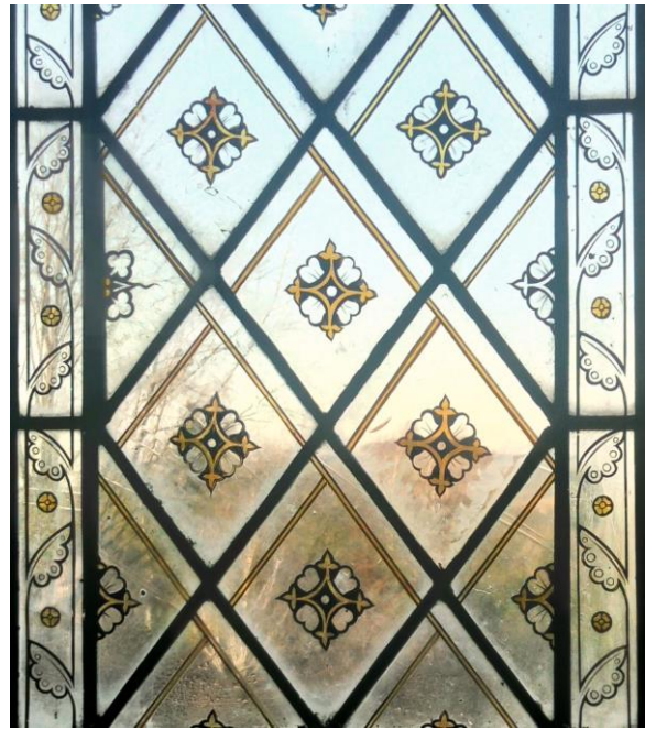
Detail: window nV light b after restoration with new painted pieces
