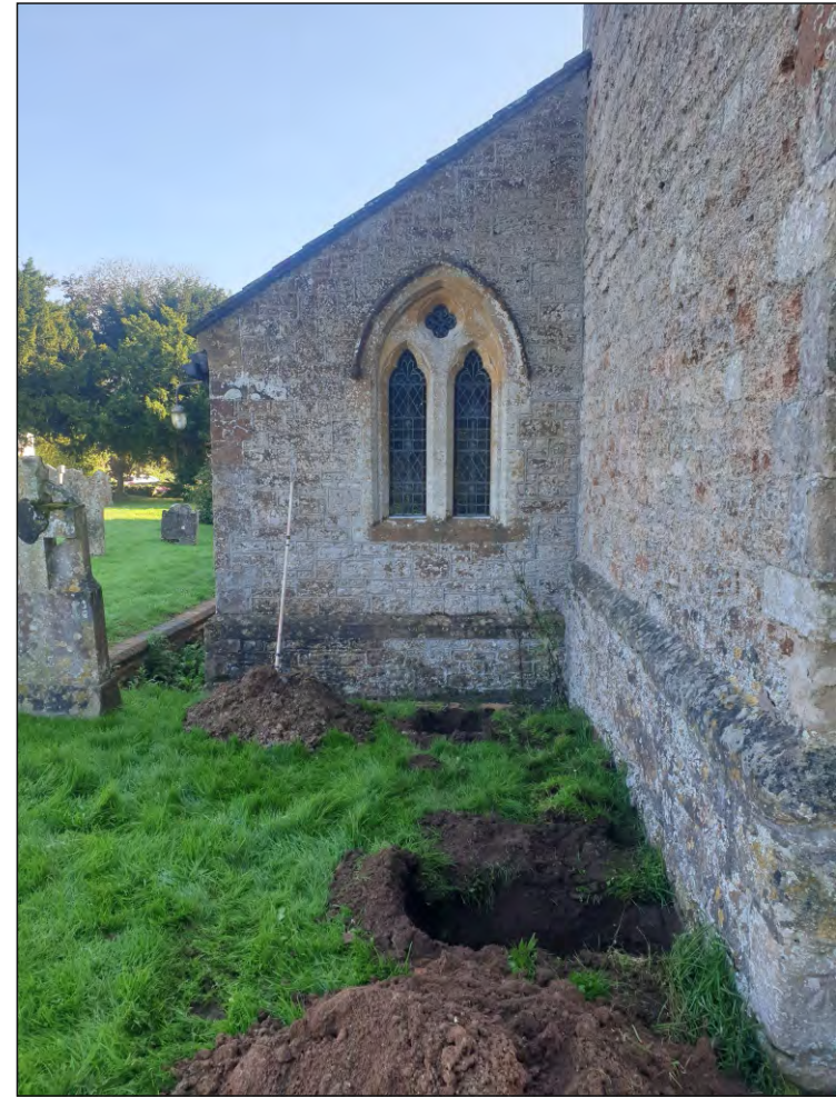
Pl. 2 General view access pits 7-8. Looking east.
