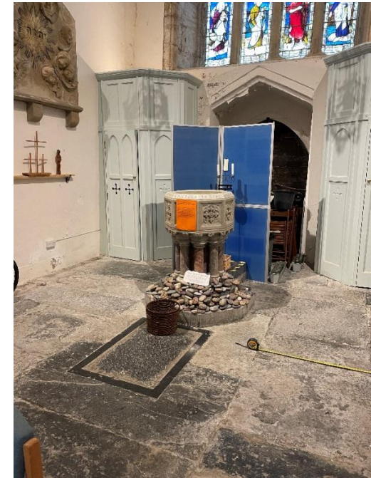
Fig 2: View of current use within the tower shows existing painted timber panelled storage cupboards to either side of the west door with a stained glass west window visible above. Stone slabs including a central ledger are seen on the floor under the font set on a stone plinth, and the existing stone monument is seen set into south wall of tower (part of the Grinling Gibbons monument).
