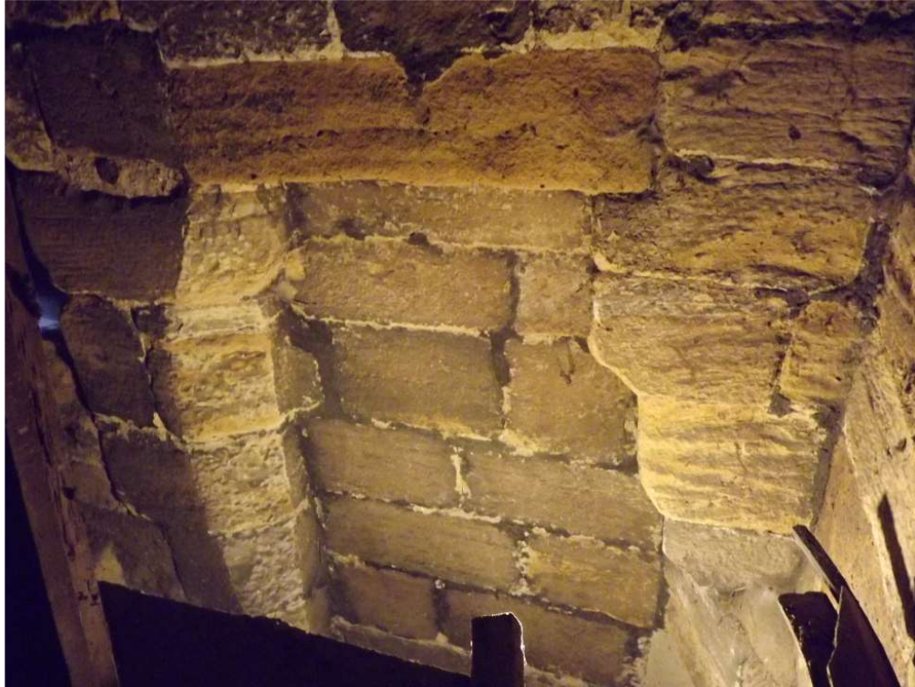
Plate 10. Probable blocked opening in south elevation
