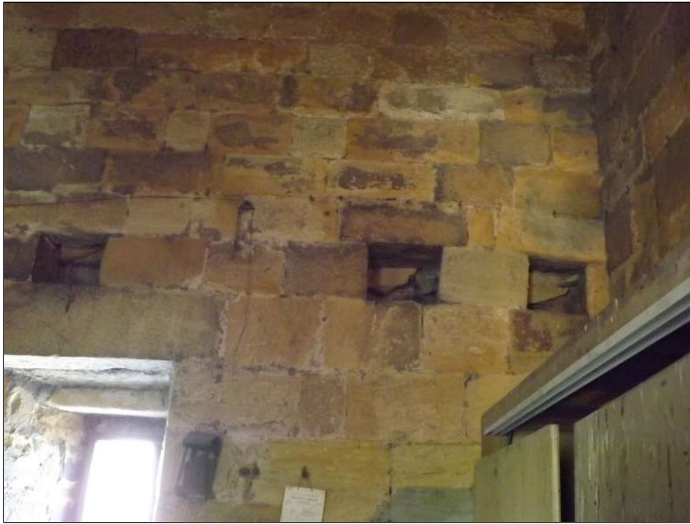
Plate 3. Joist holes in east elevation, note worked stone in 2 nd from right and slope of the right hand socket
