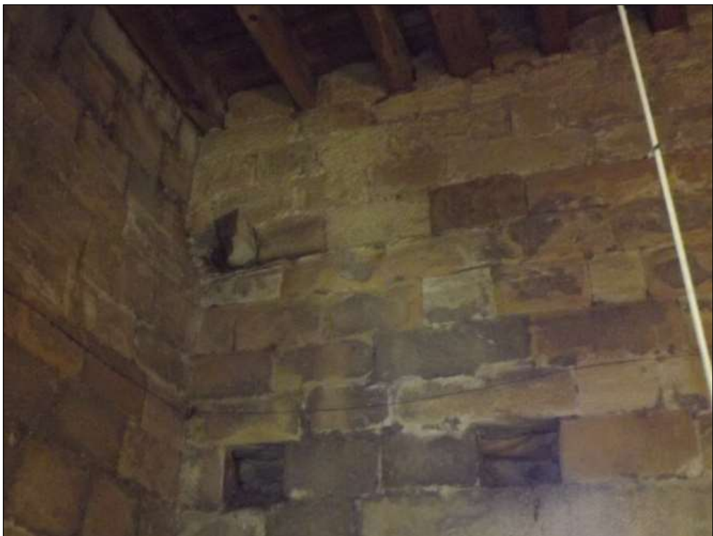
Plate 4. Timber baulk in east elevation, note change in stonework above baulk
