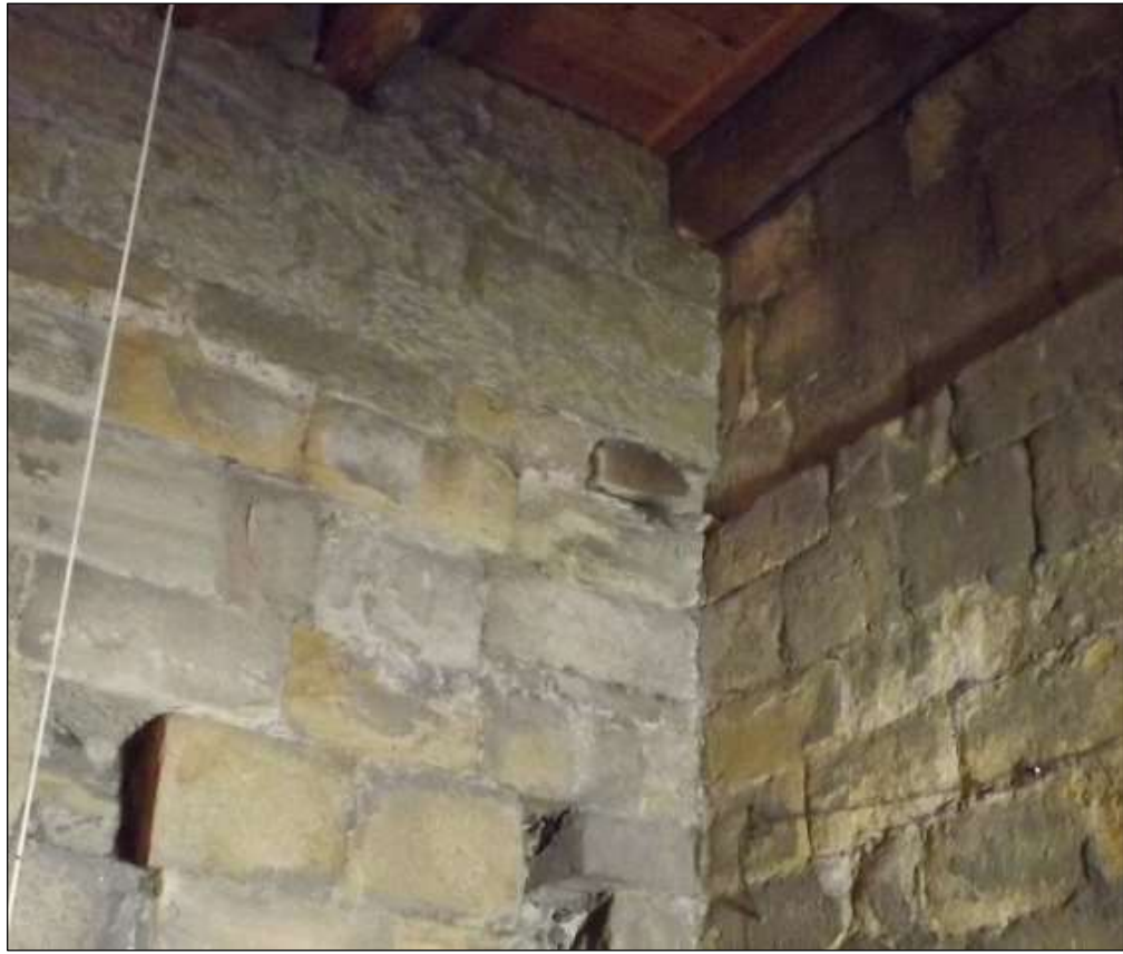
Plate 5. Timber baulk in west elevation and note change in stonework
