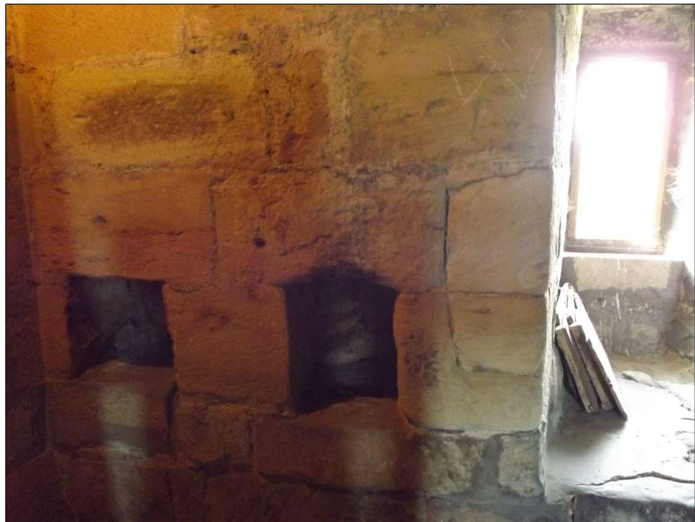
Plate 6. Lantern niche & irregular stonework in window reveal in W elevation
