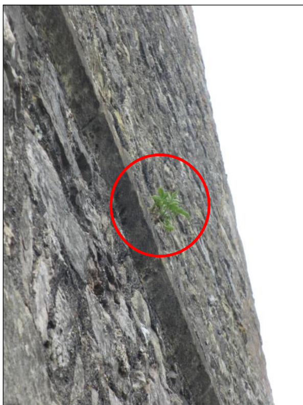
Top left : The typical condition of the stonework and failing pointing to the middle stage (west).
