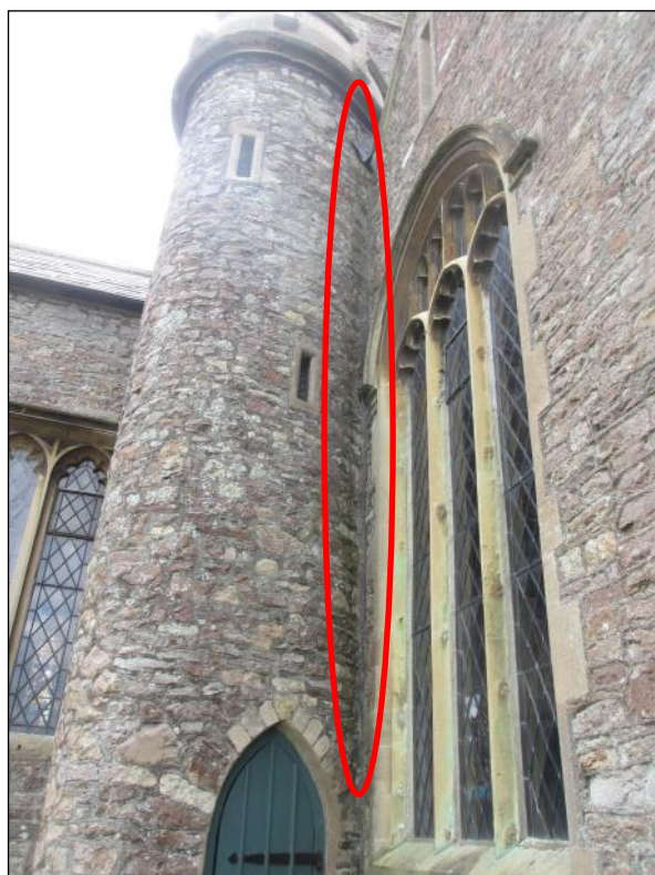
Top left : The typical condition of the stonework and failing pointing to the middle stage (west).
