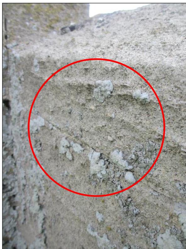
Lower left : The lead shows the extent of general erosion to the surface of the stone.
