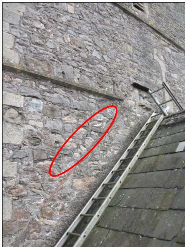
Top left : Extensive mortar loss from the stonework to the east face for of the tower. Lower left : Damaged and missing stone louvres on the south side. Top right : Two section of string course on the north side are in poor condition. Lower right : Loose masonry along the former roof line.
