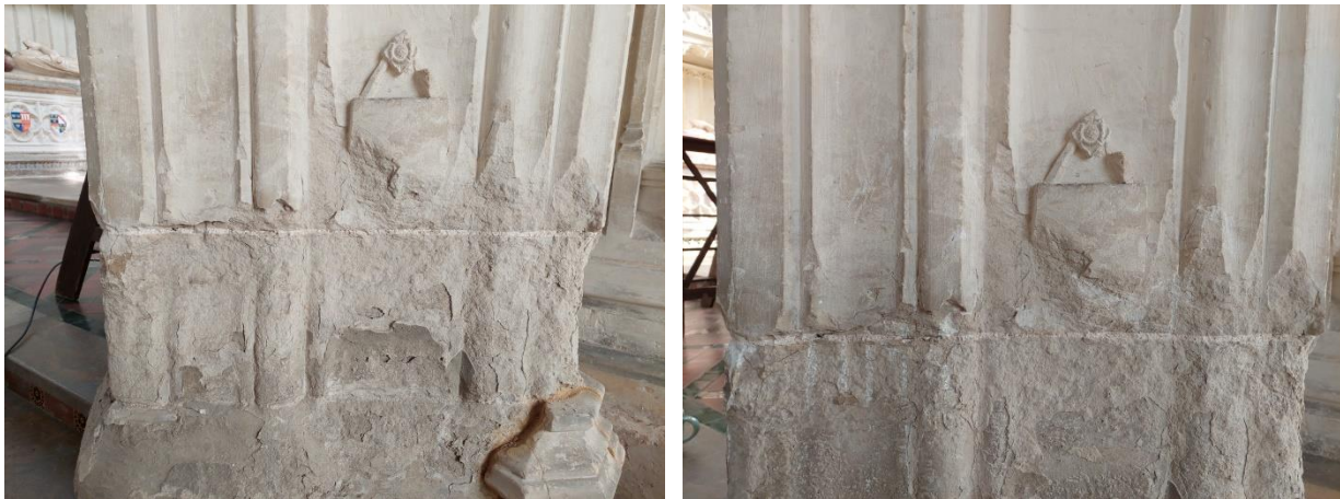
Plates 23 and 24: Carving details before and after being grouted on column west of monument
