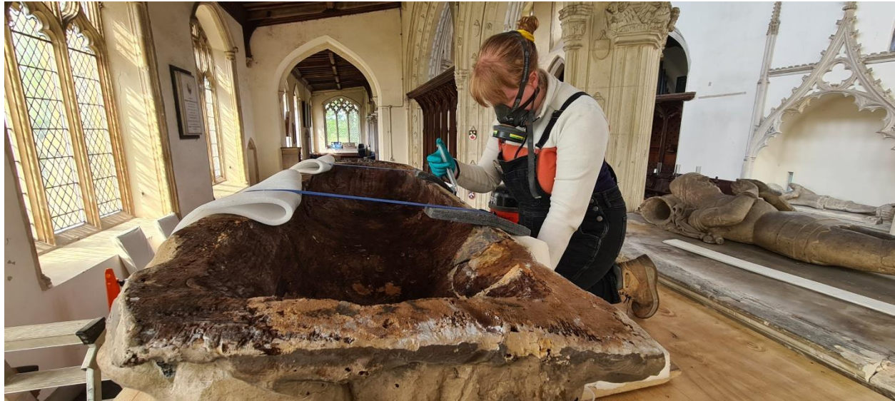
Plate 10: Katherine de la Pole being injected with Constrain.
