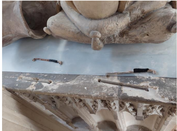
Plate 13 and 14: Rusting cramps on top of the tomb chest being replaced with stainless steel
