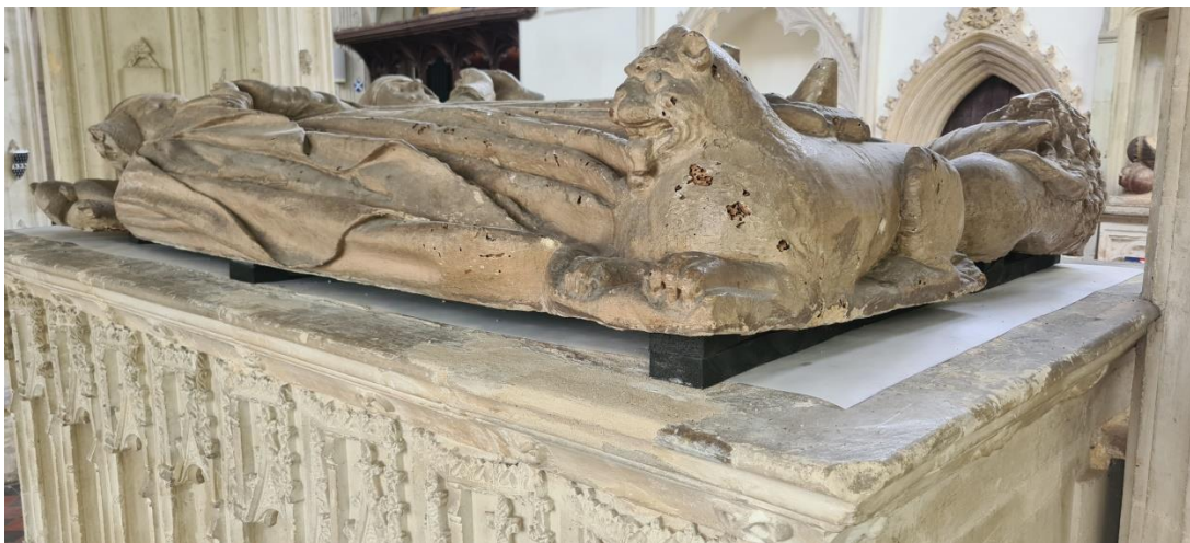
Plate 27: Repair to south side of cornice and replaced cramps
