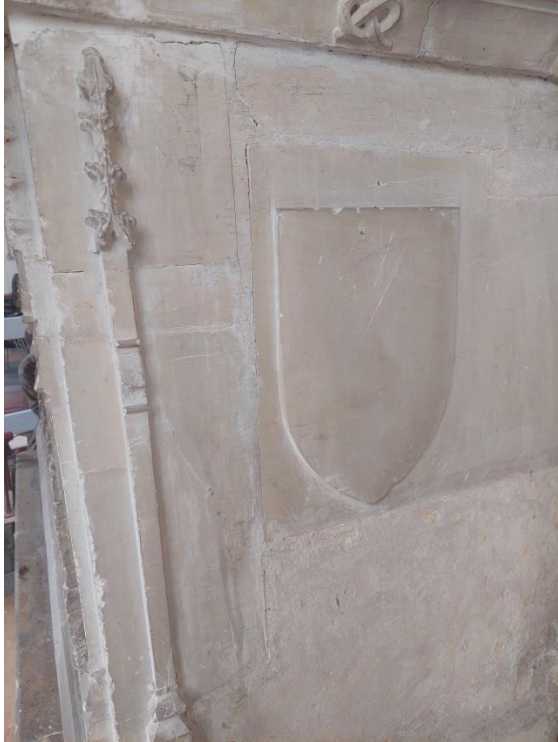
Plate 33: Graffiti removed with historic graffiti arch still remaining
