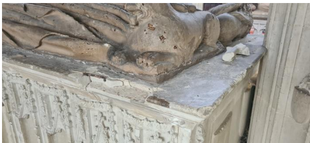
Plates 17 and 18: Before and after the re-attachment of loose indent
