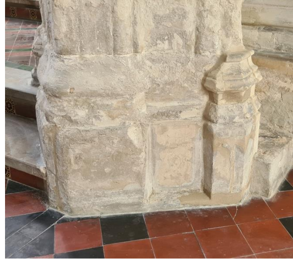
Plate 26: Mortar repairs to re-attached section
