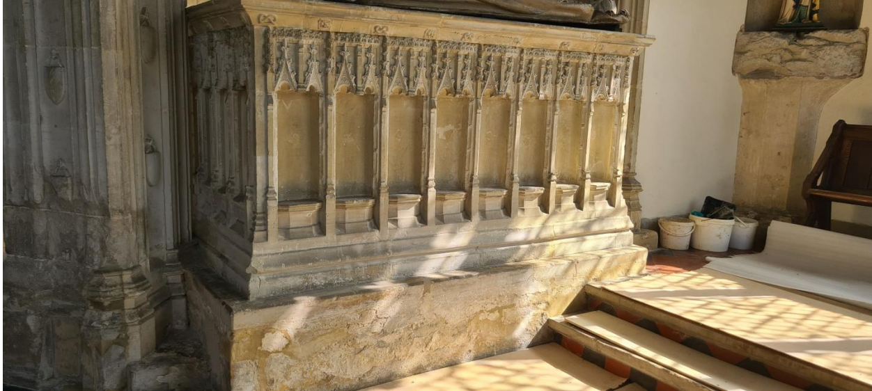
Plate 16: Mortar repair after removing historic iron fixings
