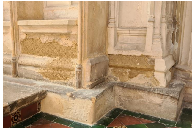
Plates 28 and 29: During and after lime putty repairs to base of monument (north side)
