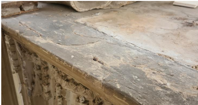
Plate 13 and 14: Rusting cramps on top of the tomb chest being replaced with stainless steel
