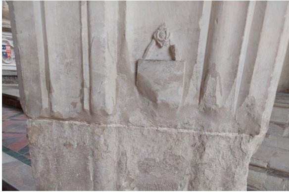
Plate 25: Mortar fillet to carved details on column
