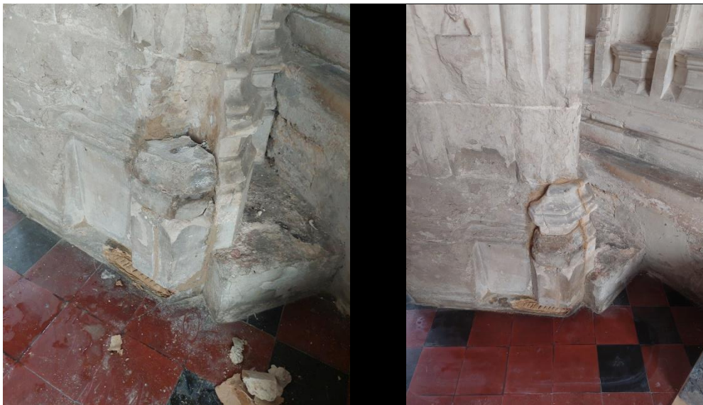
Plates 19, 20, 21 and 22: Column section before removing, and during reconstruction including found section from top of tomb chest
