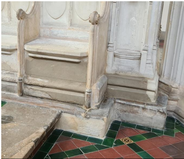
Plates 28 and 29: During and after lime putty repairs to base of monument (north side)
