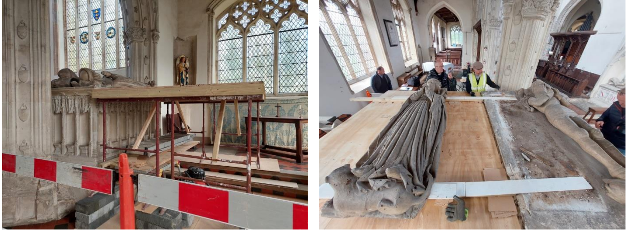
Plates 4 and 5: Temporary platform and Katherine de la Pole being moved by Teflon skids
